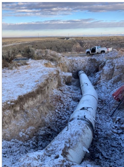
Mainline Pipe Installation: Photo taken looking north along the Old Dam Road, towards the Historic Teton Dam, where the 36” pipe was tied into the 42” pipe.
