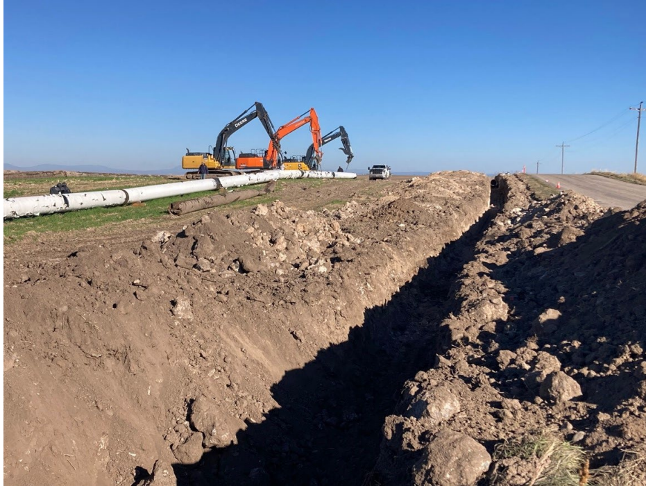
Mainline Pipe Installation: Photo taken looking north along the Old Dam Road, towards the Historic Teton Dam, where the 36” pipe was tied into the 42” pipe.
