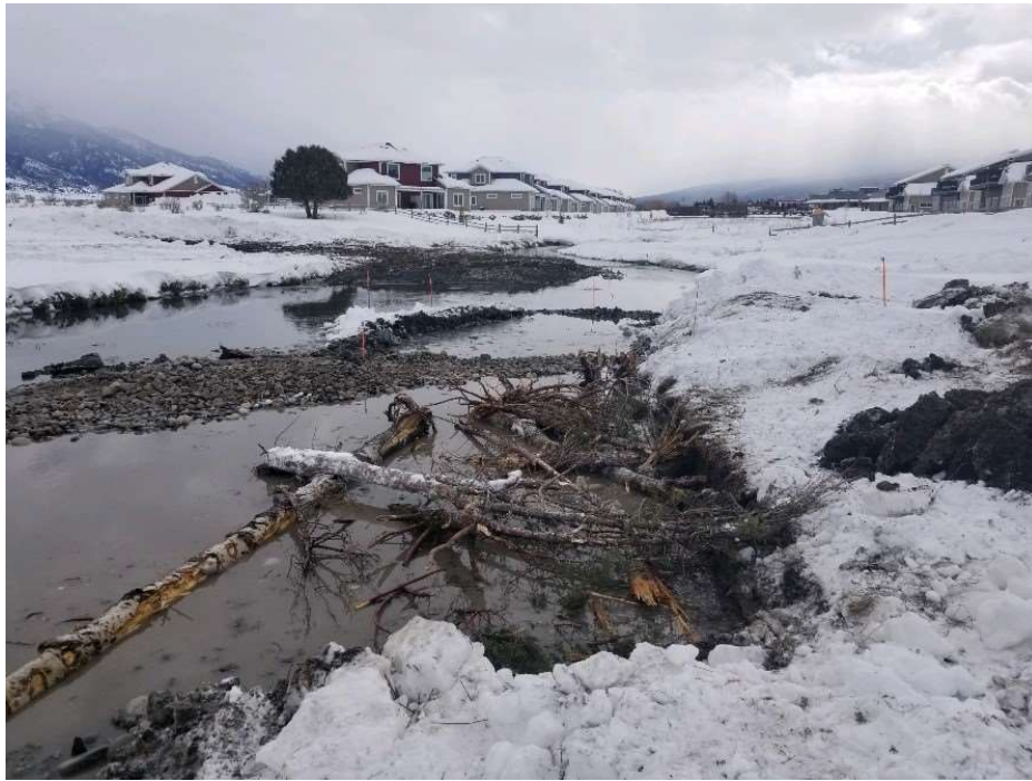
Photo 1. Phase 2, during project implementation. Newly constructed large wood debris log structure.
