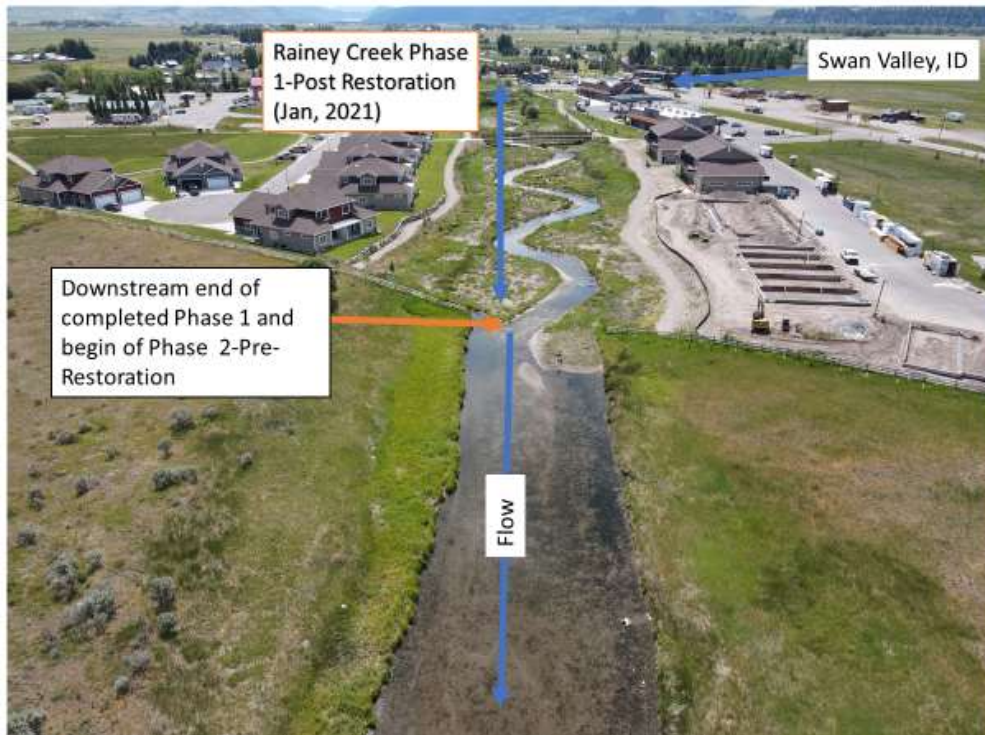
Photo 3. Pre-Restoration. Top of Phase 2 facing upstream into recently completed Phase 1.
