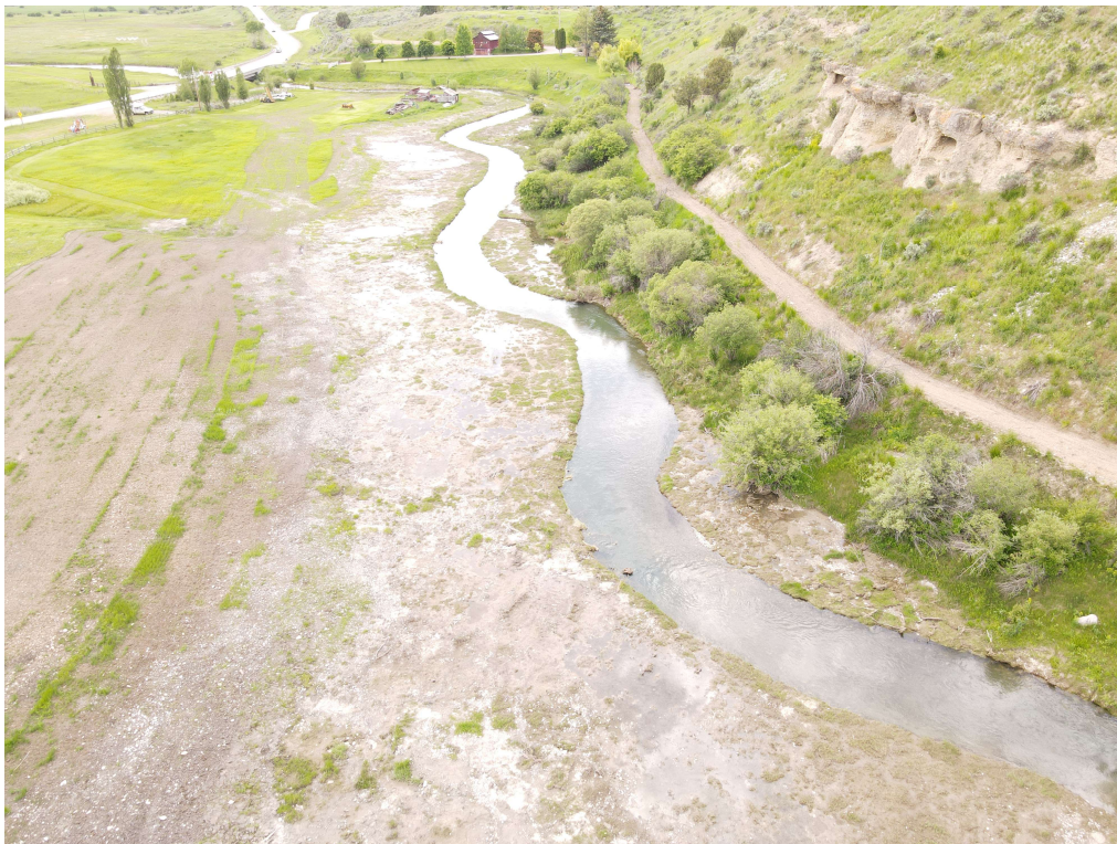
Photo 8. Post Restoration-Phase 2. Facing downstream, Notice narrower channel with improved sinuosity and habitat (large wood added).
