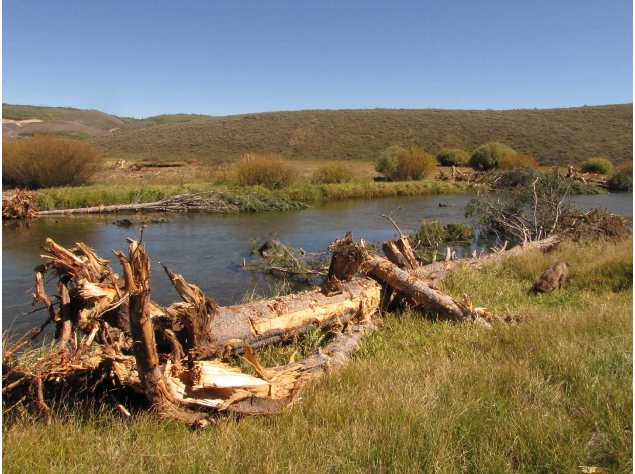
Figure 5. In stream wood treatment constructed with whole trees.
