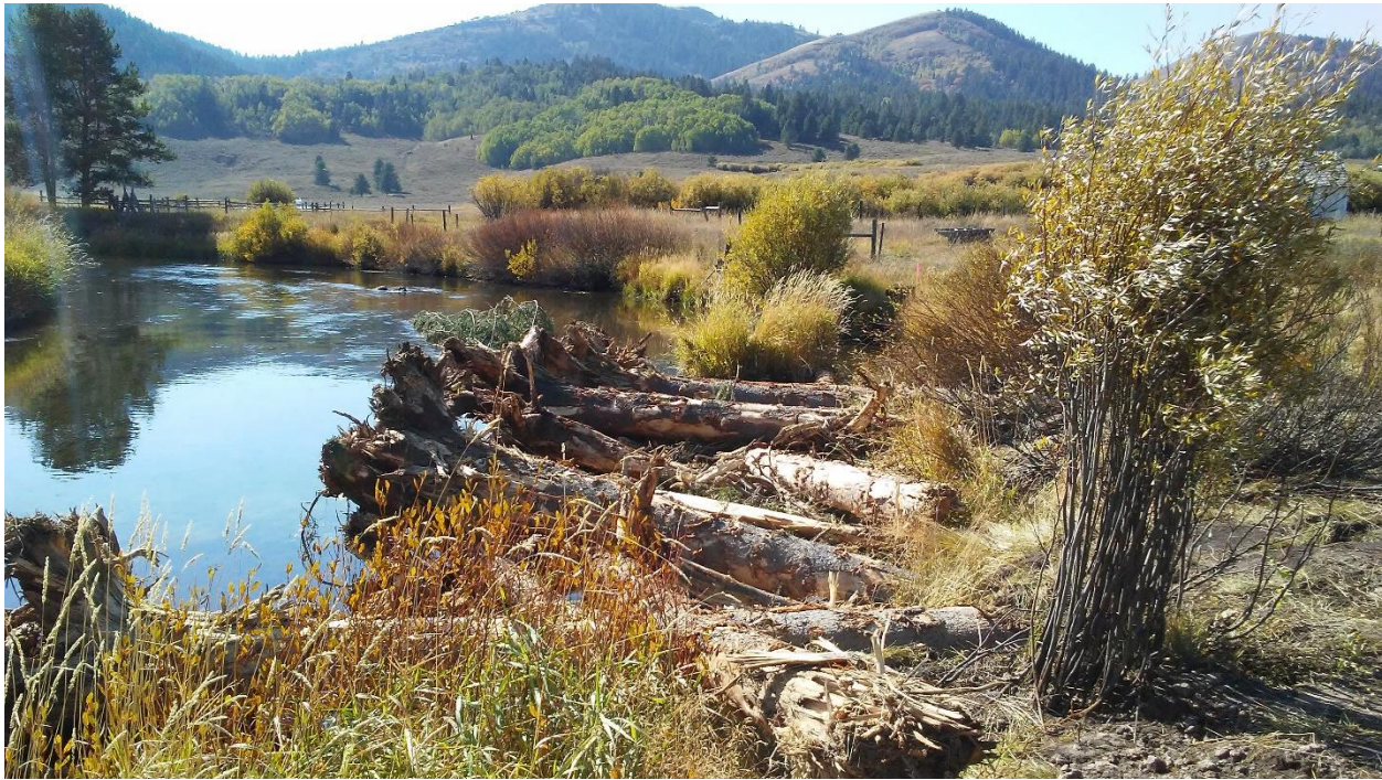
Figure 9. Transplanted willow clumps to jump start willow recruitment increasing shading and providing natural bank stabilization.
