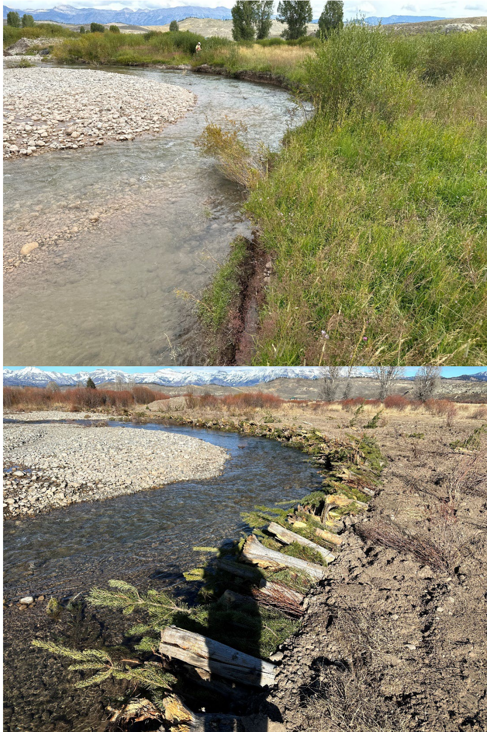
Photo Set 9. Steep eroding bank with poor fish habitat (above), regraded bank with logs with rootwads, brush, and willows (below).
