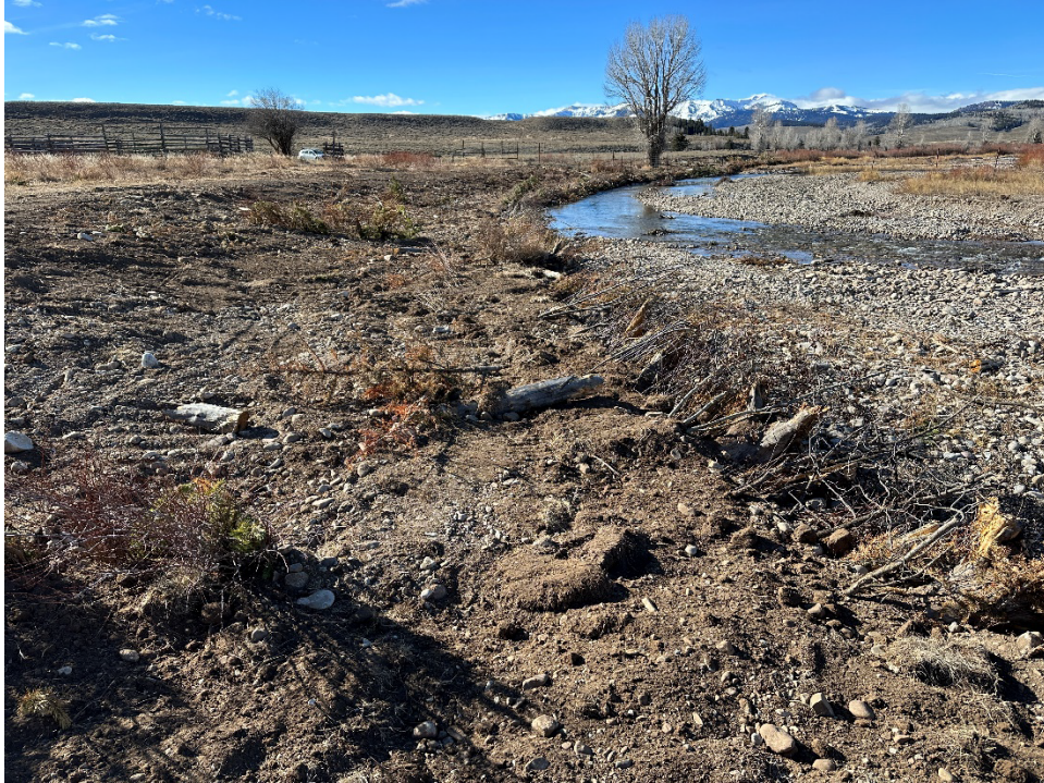
Photo Set 7. High, eroding outside banks lacking floodplain connectivity (above); brush bank structure with floodplain bench and floodplain roughness treatment (below).
