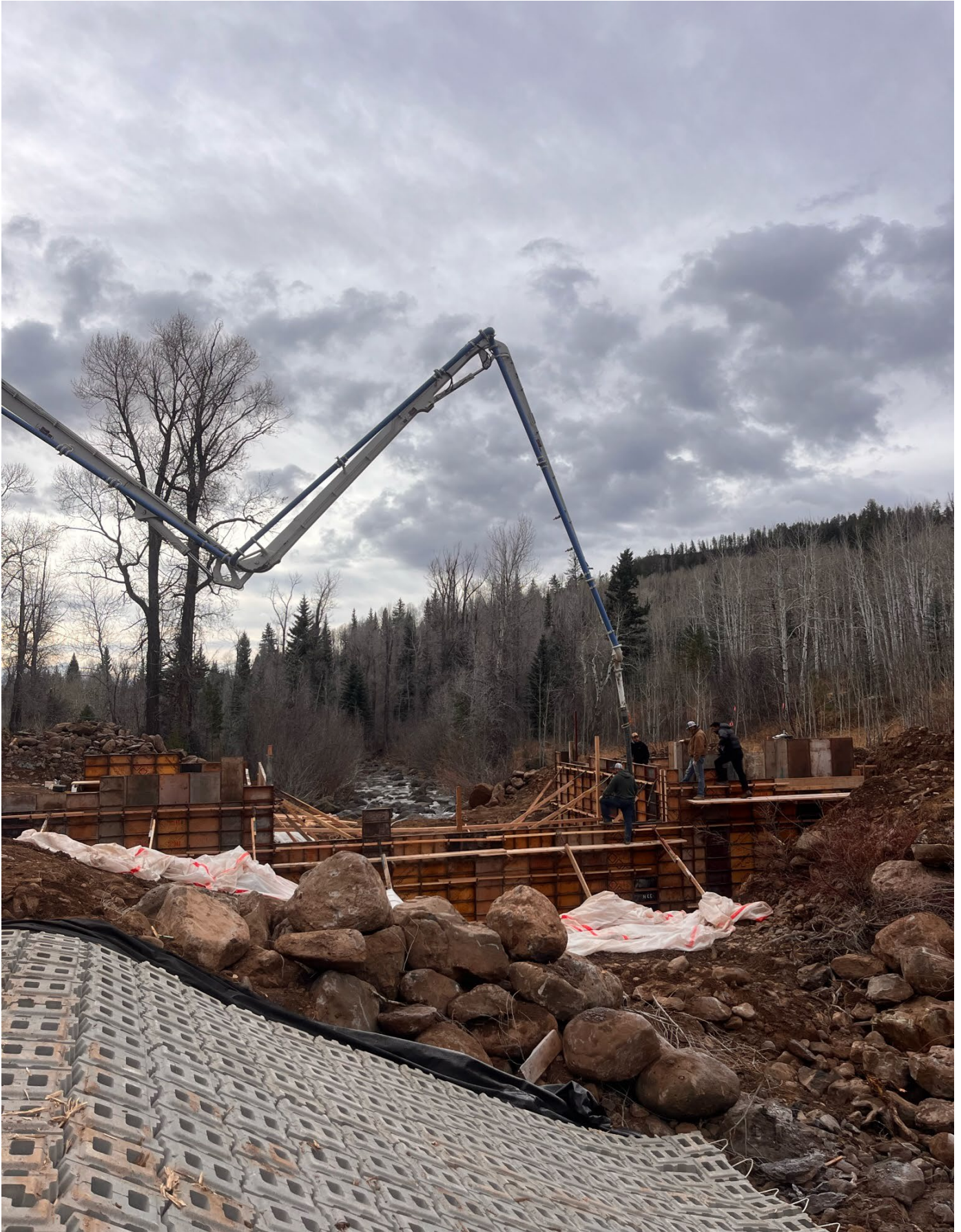
Concrete forms and pour for fish barrier
