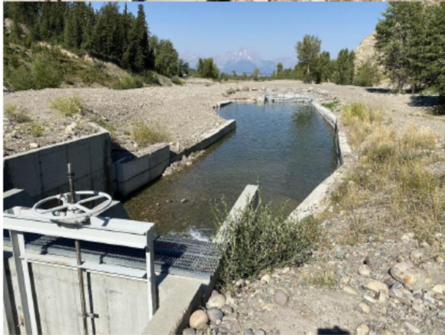
Photo Set 11. Previous headgate and sediment basin (above), expanded sediment basin and new fish screen at far end (below).
