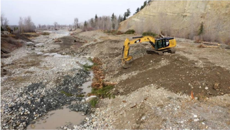
Photo 1. Bank stabilization structures using a combination of wood, rock, resloping, and erosion fabric were installed in November 2021.
