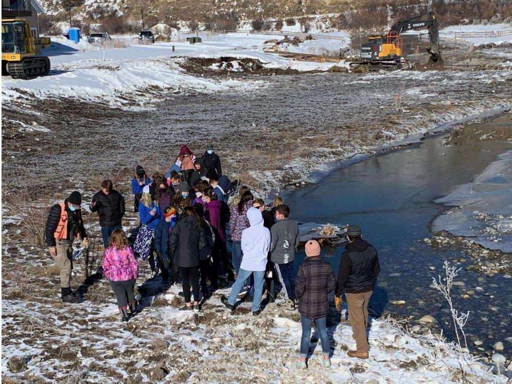
USFS Hydrologist (Louis Wasnieski) providing a tour of the Bridge to Bridge - Phase 1 Rainey Creek Restoration project to local elementary students.
