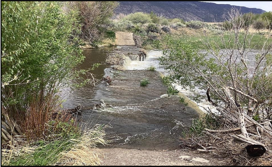
Photo Point: Before #1 File Name: 1 Pre Project East Channel Across Diversion.png Photo Description: East channel looking directly across the diversion towards the west. Photo Date: 05/18/2020
