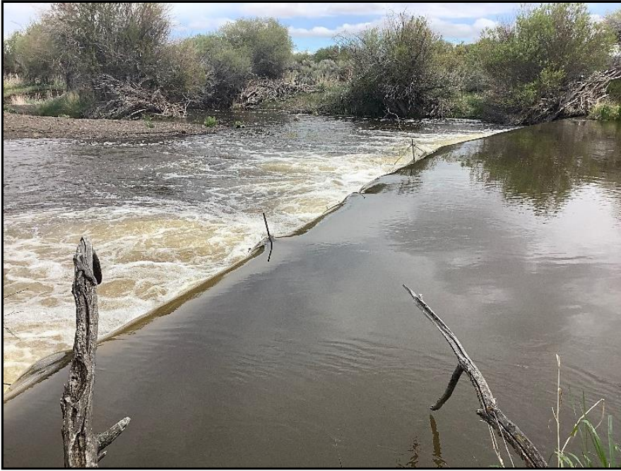
Photo Point: Before #4 File Name: 4 Pre Project West Channel Across Diversion.png Photo Description: West channel looking across the diversion facing north Photo Date: 05/18/2020
