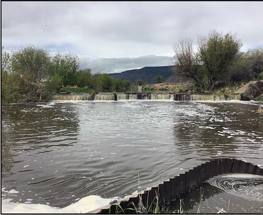
Photo Point: Before #2 File Name: 2 Pre Project East Channel Below Diversion.png Photo Description: East channel looking upstream below the diversion facing south/southwest Photo Date: 05/18/2020
