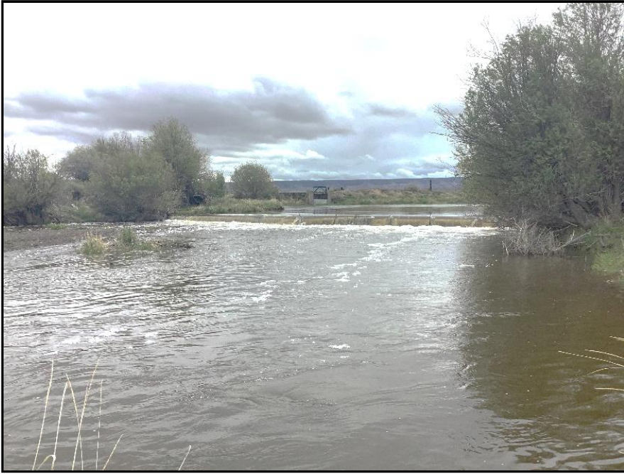
Photo Point: Before #5 File Name: 5 Pre-Project West Channel Below Diversion.png Photo Description: West channel looking upstream below the diversion facing east Photo Date: 05/18/2020
