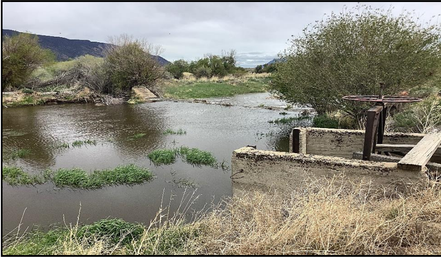
Photo Point: Before #3 File Name: 3 Pre Project East Channel Above Diversion.png Photo Description: East channel looking downstream above the diversion facing north/northwest Photo Date: 05/18/2020
