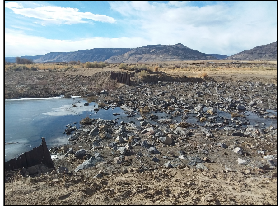
Photo Point: After #1 File Name: 1 Post Project Looking Across Old Weir .jpg Photo Description: Relict Weir Project looking across the stream at the location of old weir facing west Photo Date: 01/21/2021
