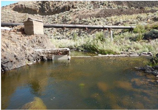
Figure 2. Distant (left) and close-up (right) views of the Middle Diversion intake headwall with road sign in front of the intake for controlling flow into the pipeline.
