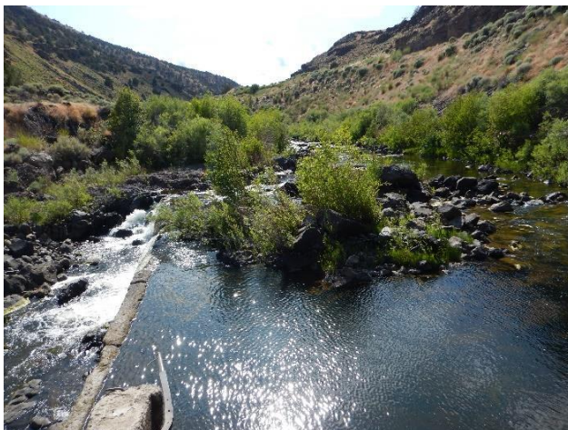
Figure 3. A view across the Middle Diversion weir from river-left showing the bedrock outcrop on the left bank (left), and a view of coarse bed materials upstream from the weir (right).
