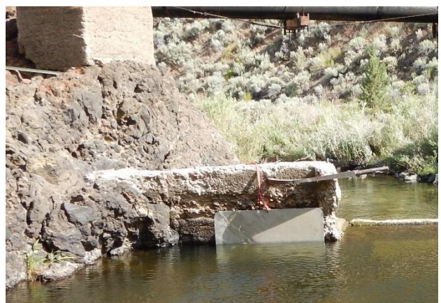
Figure 2. Distant (left) and close-up (right) views of the Middle Diversion intake headwall with road sign in front of the intake for controlling flow into the pipeline.
