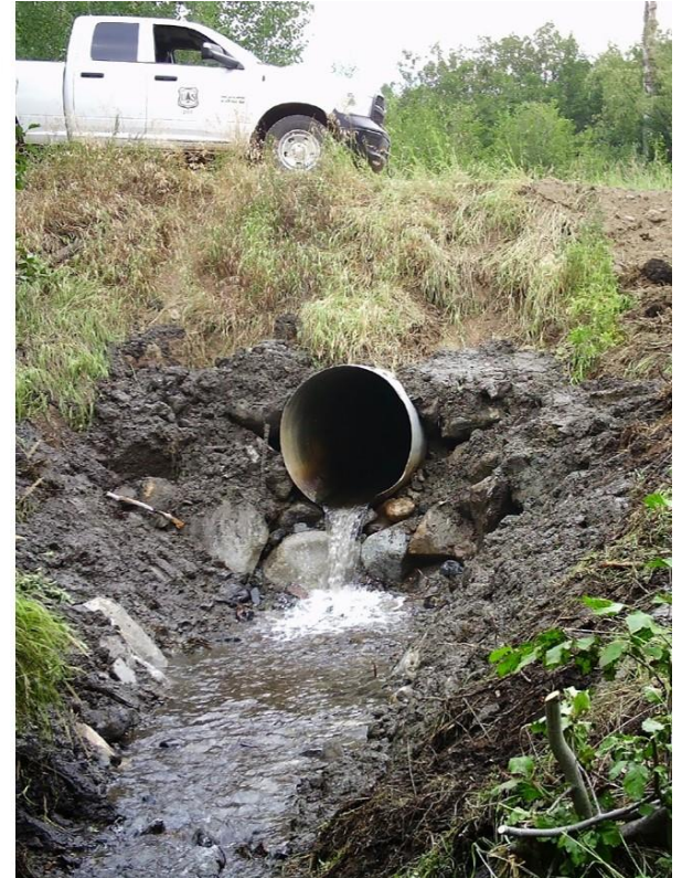
Photo 5. The middle Eagle Creek culvert located upstream from the Eagle Creek Camp Ground before beaver dam removal (left), after beaver dam removal (middle), and after excavation and armoring to prevent upstream invasion of nonnative fish (right).
