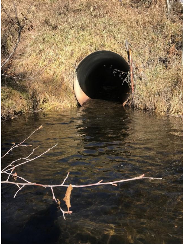
Photo 5. The middle Eagle Creek culvert located upstream from the Eagle Creek Camp Ground before beaver dam removal (left), after beaver dam removal (middle), and after excavation and armoring to prevent upstream invasion of nonnative fish (right).
