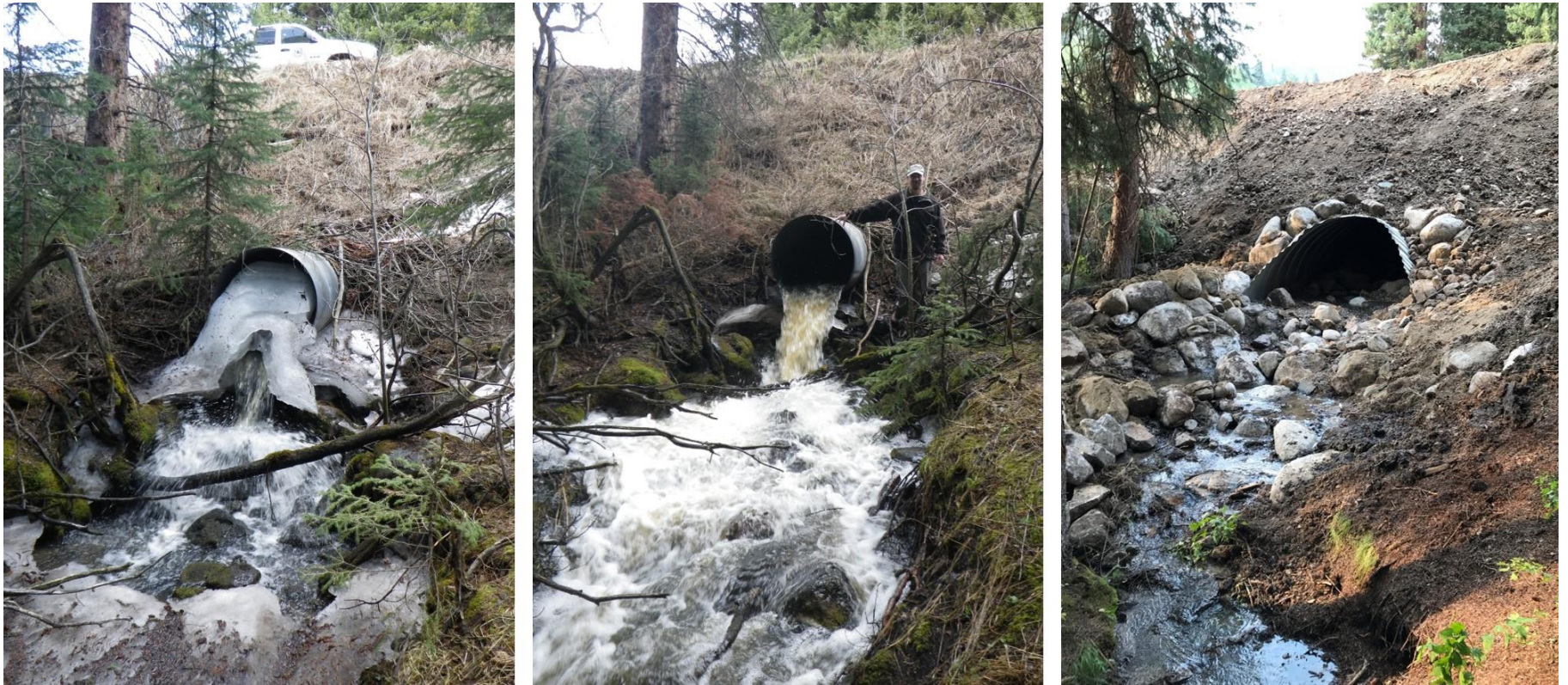
Photo 2. The Eagle Creek crossing before (left and middle) and after being upgraded to provide for aquatic organism passage (right).
