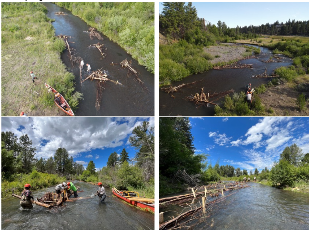
Figure 3. Willow Springs Preserve Phase I Restoration Summer 2022
