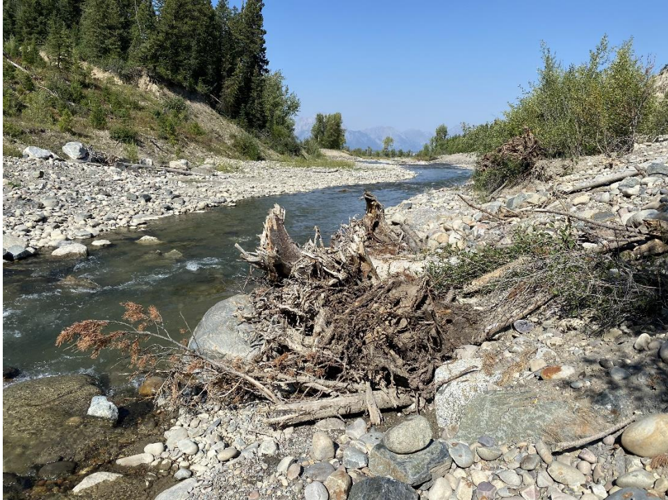
Photo Set 9. Before and after. Eroding bank (above), engineered log jam (below).
