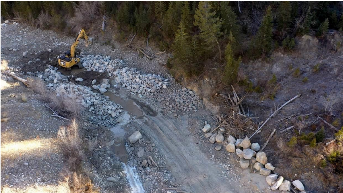
Photo 2. Large boulders were imported to create a rock ramp diversion structure in November 2021, a design expected to be much more robust than the previous diversion structure.
