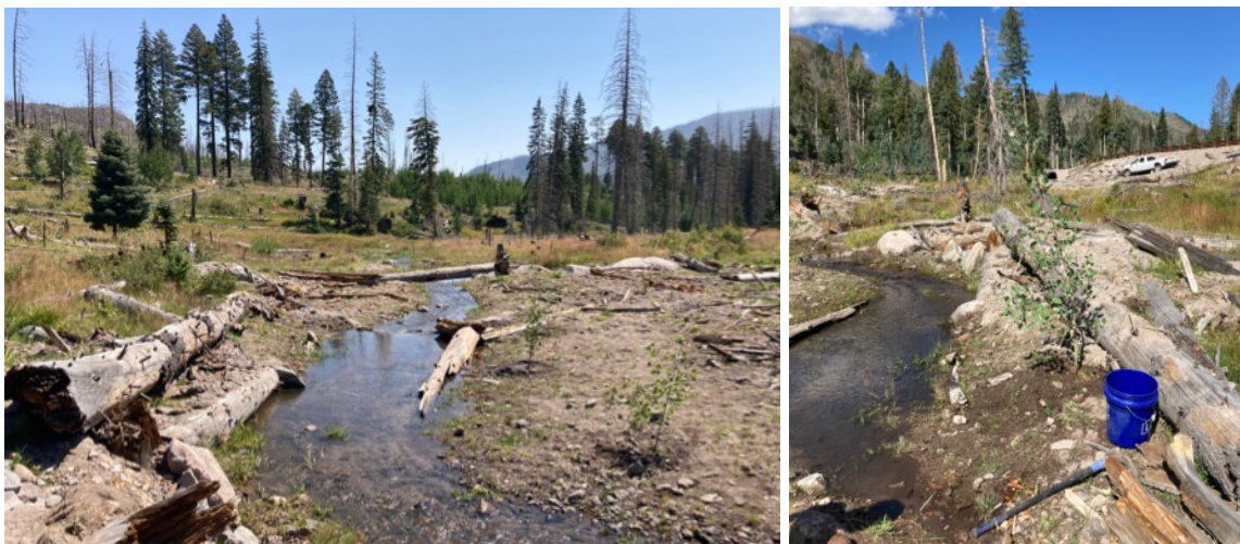
Fig. 3) A WNTI treated site that depicts toe-wood that had water redirected to undercut the log, a downstream rock vein installed to facilitate pooling, and woody debris dispersal with aspen planting to promote cover.
