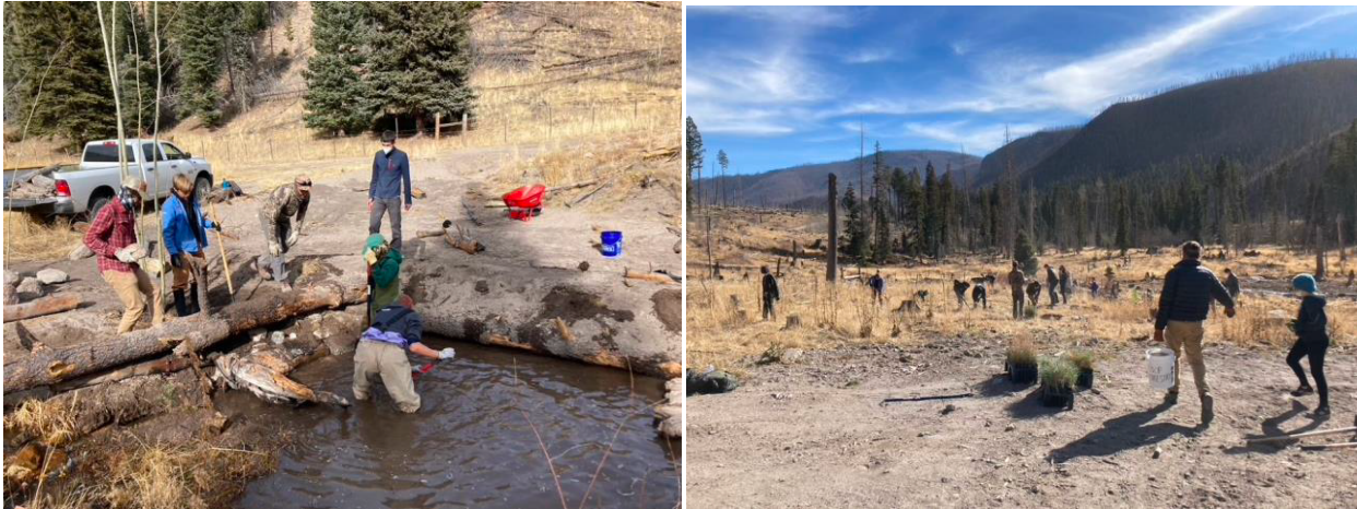
Fig.7) Outreach activities provided additional support to the successful completion of this project by integrating “toe-wood” to provide bank stability and habitat cover. Douglas fir and Ponderosa conifer seedlings were then planted in adjacent uplands, and grass plugs were sourced from adjacent vegetated areas to facilitate shading and habitat connectivity.
