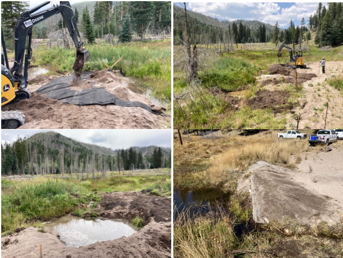
Fig. 4) Off-channel pond creation in a relic wetland historically occupied by beaver. The enhancement created four off-channel ponds that will provide freeze resistant habitat for trout, while increasing surface and subsurface water storage to provide habitat resilience to drought.
