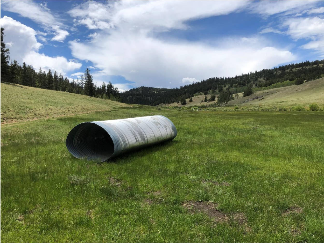
Photo 6. Fish passage culvert (Prior to being installed by private landowner).
