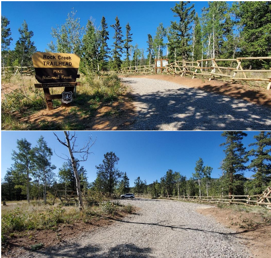
Photo 2. Completed buck and rail fencing around the parking area.
