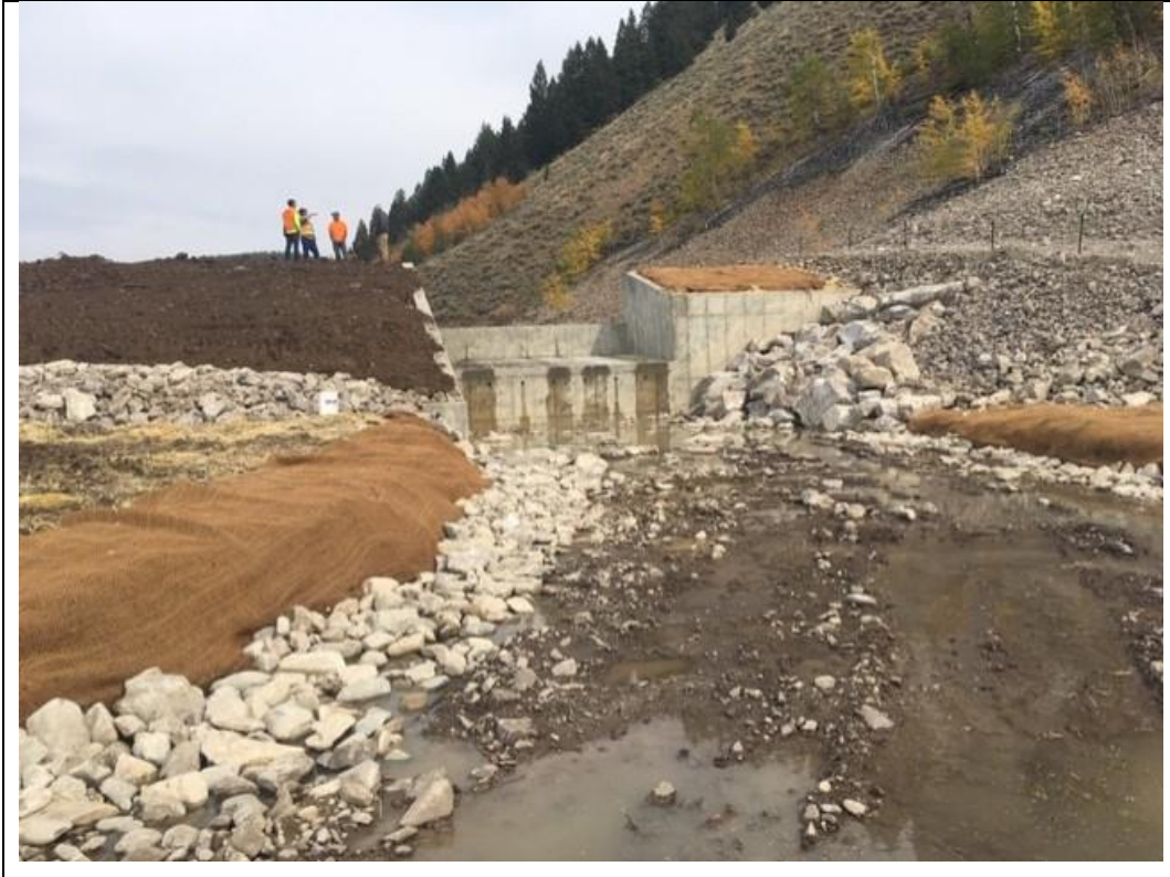
With the side-walls and barrier completed and the backfilling finished, the stream channel is reestablished prior to returning flows. Photo: Matt Jaeger, Montana Fish Wildlife and Parks
