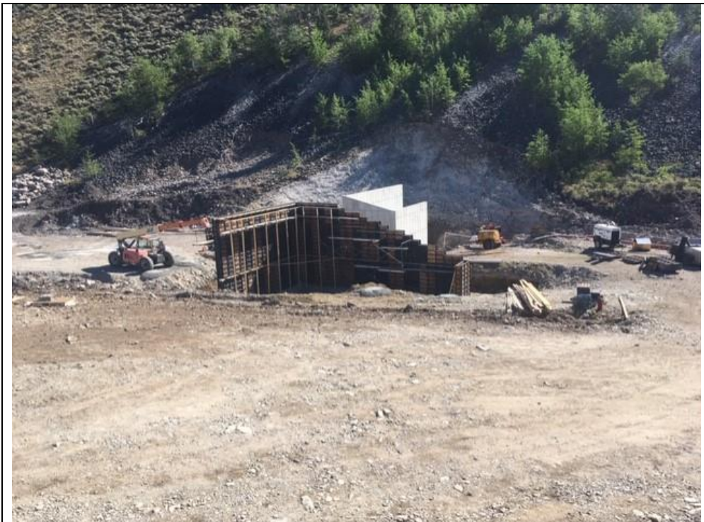
Forming up the walls following the completion of the foundation. Photo: Matt Jaeger, Montana Fish Wildlife and Parks.
