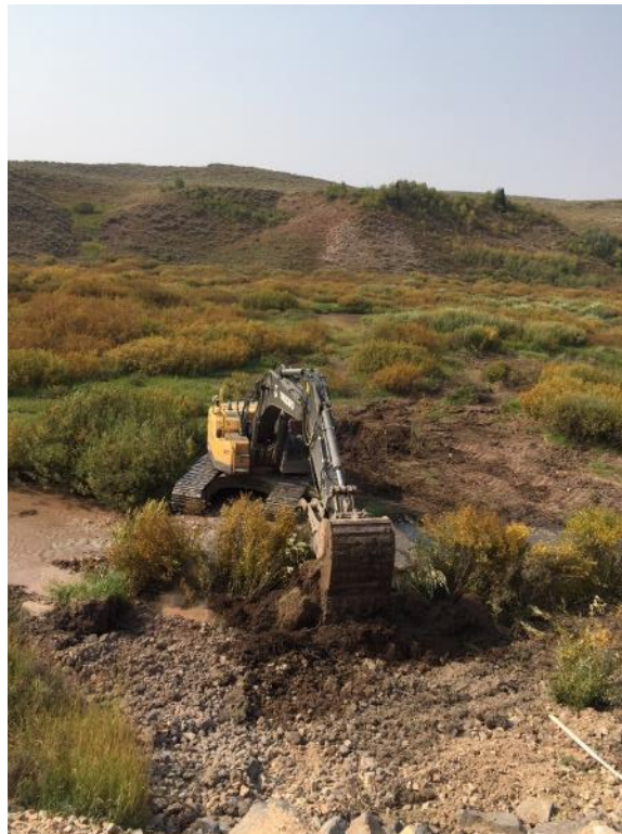
Tara Hicks, co-owner/operator of Rockin' T Construction, transplanted sod and whole willow clumps to build and rapidly revegetate new stream bank in 2017.
