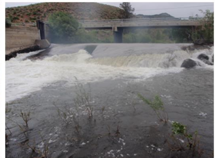
Left: Town Diversion – Southeast view demonstrating summer low flows. The diversion is a complete fish passage barrier due to vertical drop over the structure. Center and Right: In the Spring, high velocities also create a complete barrier to fish passage.
