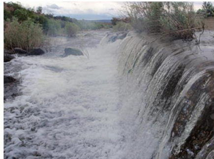
Left: Town Diversion – Southeast view demonstrating summer low flows. The diversion is a complete fish passage barrier due to vertical drop over the structure. Center and Right: In the Spring, high velocities also create a complete barrier to fish passage.
