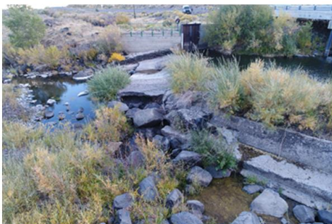
Left: Town Diversion – Southeast view demonstrating summer low flows. The diversion is a complete fish passage barrier due to vertical drop over the structure. Center and Right: In the Spring, high velocities also create a complete barrier to fish passage.
