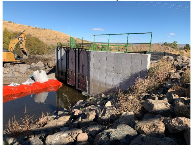
Exhibit 2: Headworks, Safety Rails, Headwall
