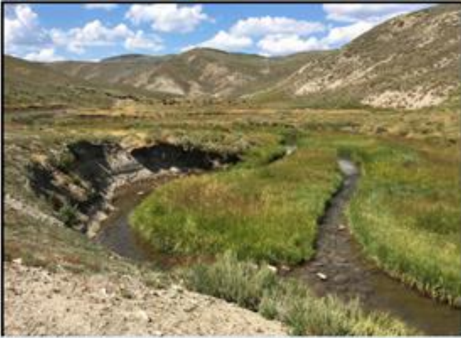
Before/after of a channel reconstruction to reduce high near-bank stress and erosion; a backwater in the former river right channel now provides juvenile fish rearing habitat.
