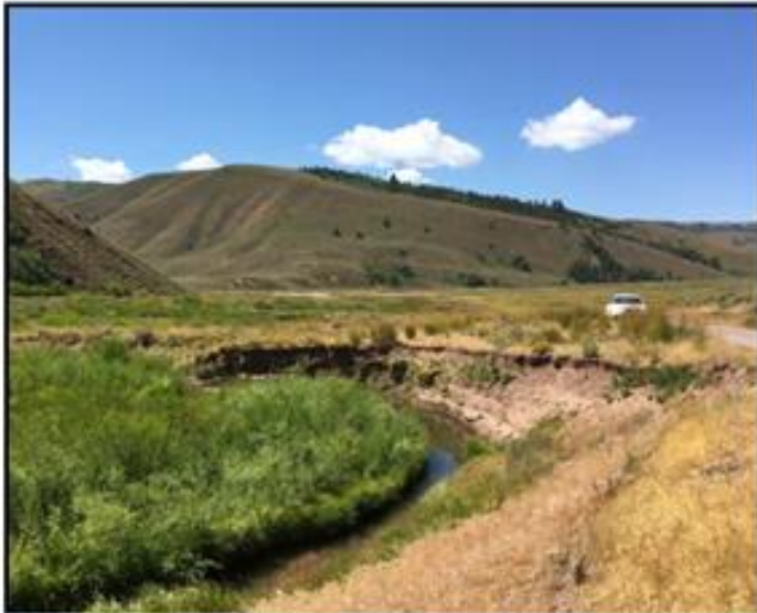
Photos from before (left) and after (right) bank re-sloping and construction of a bankfull bench to reduce sediment inputs from a large eroding bank.
