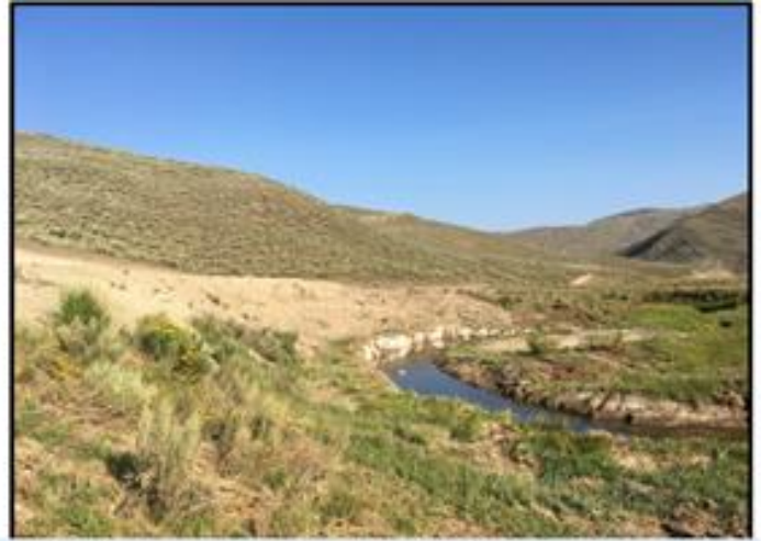
Before/after of a channel reconstruction to reduce high near-bank stress and erosion; a backwater in the former river right channel now provides juvenile fish rearing habitat.
