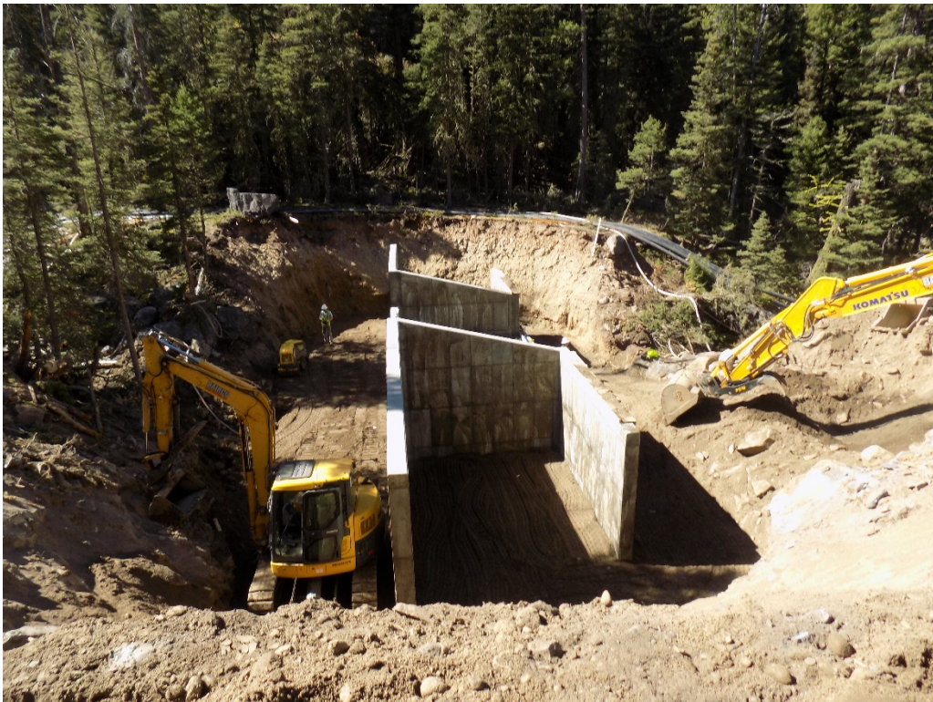
Figure 4. Fish movement barrier under construction – September 18, 2019.
