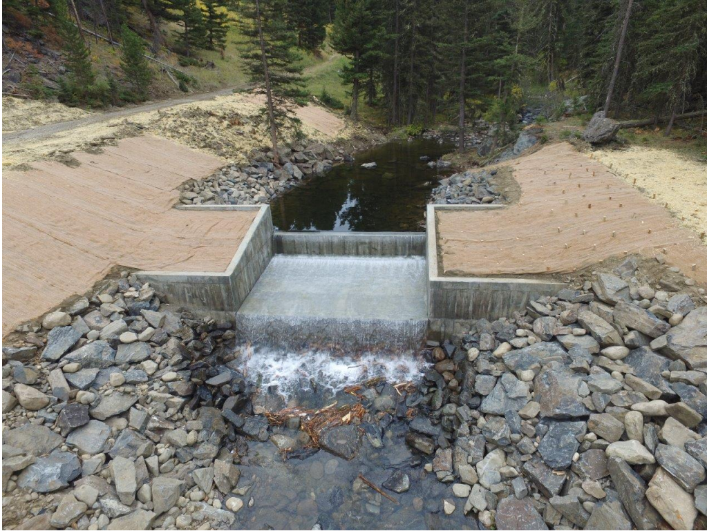
Figure 5. Completed fish movement barrier – September 28, 2019.
