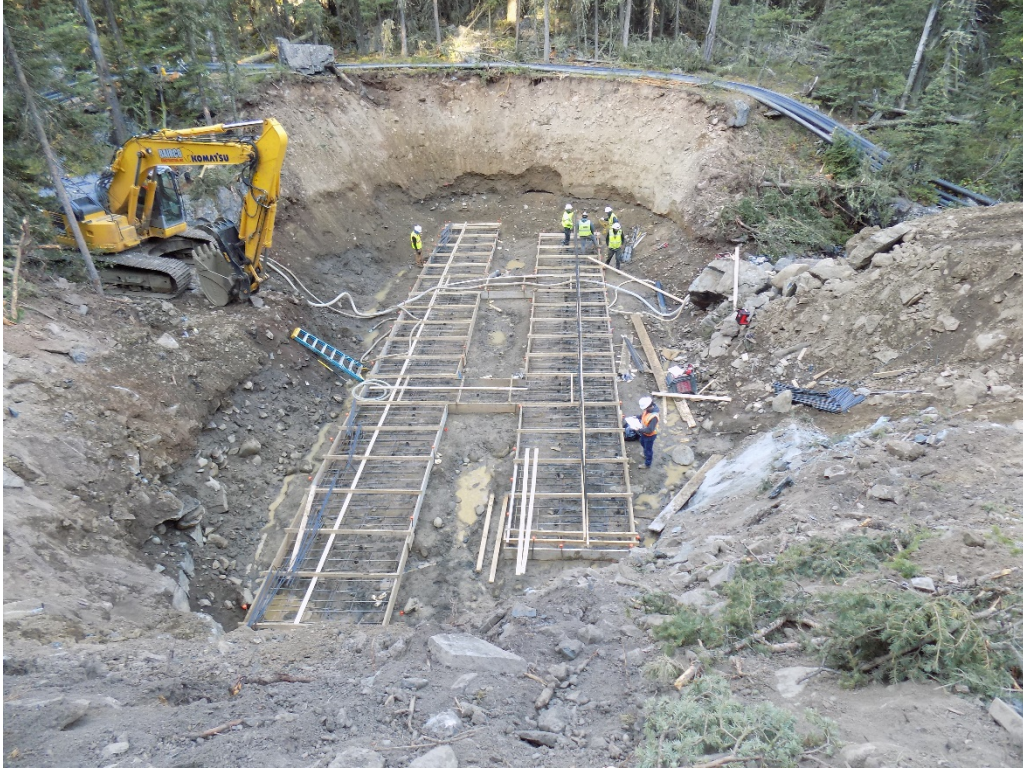
Figure 3. Fish movement barrier under construction – Sept 4, 2019.
