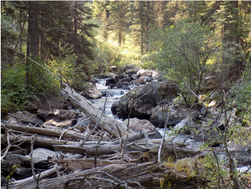
Figure 2. NF Spanish Creek fish movement barrier site – August 14, 2019.
