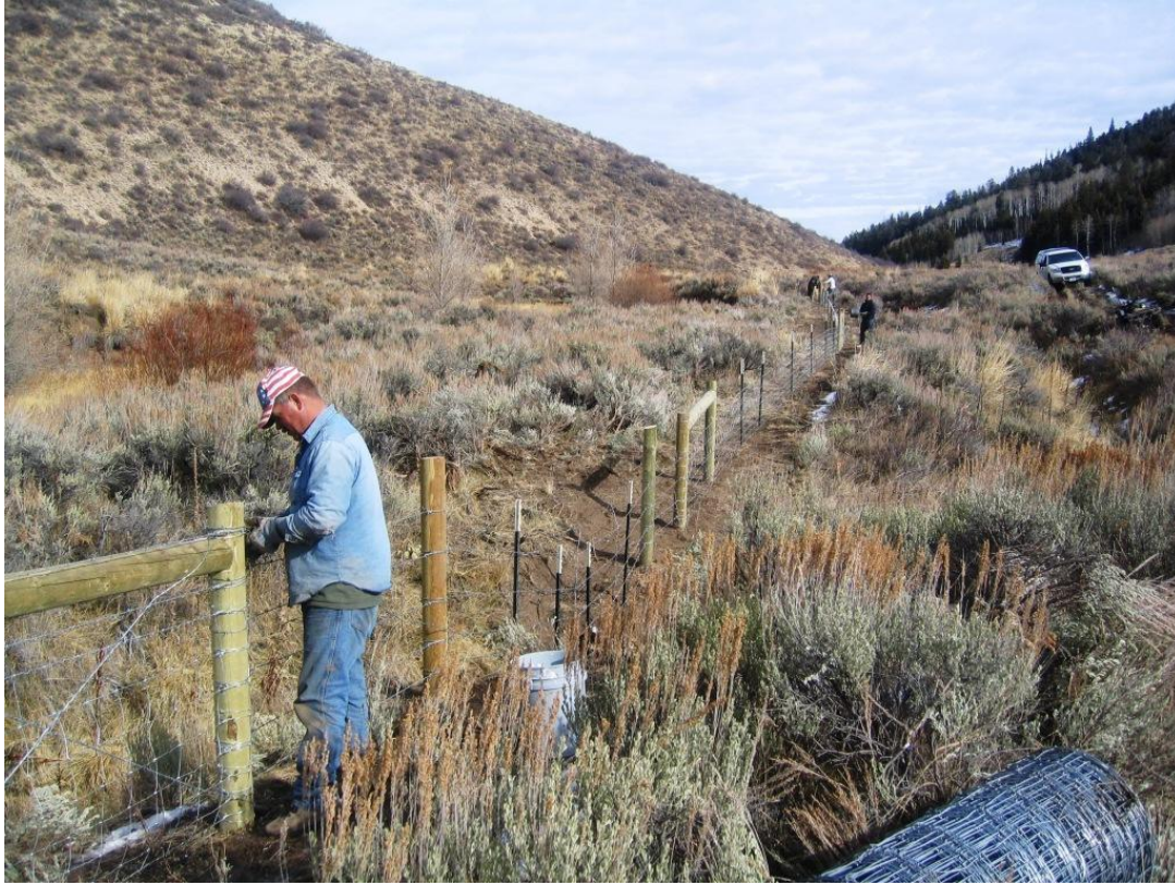
Constructing the new fence
