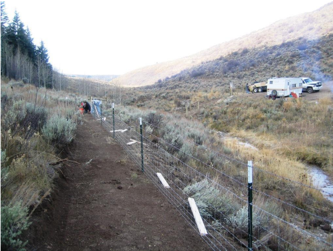
New Fence (putting up the stays) Upper Exclosure
