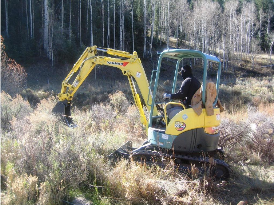
Constructing the new fence line
