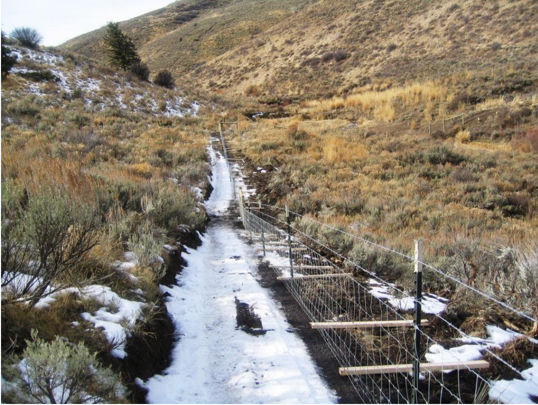
New Fence (just need the stays put up) Lower Exclosure
