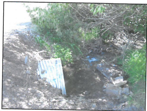
Figure 3. Hutch Creek, post-project. New culvert is larger and more appropriately placed.
