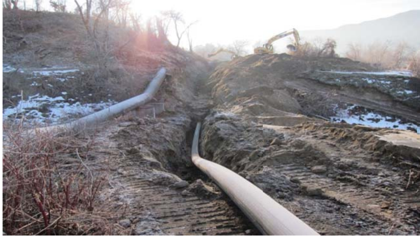
On the left- 3 foot steel pipe from the old gravity canal system, on the right is the new 14 inch HDPE pipe being installed.
