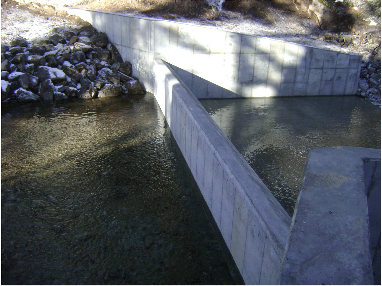
Figure 8. The bypass pipe has been plugged, and water is becoming impounded behind the barrier.
