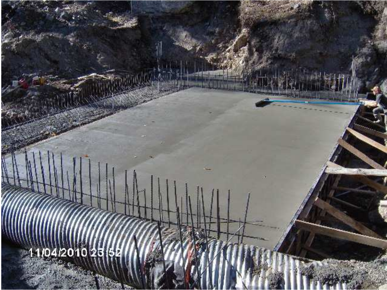
Figure 5. Concrete apron and bypass pipe
