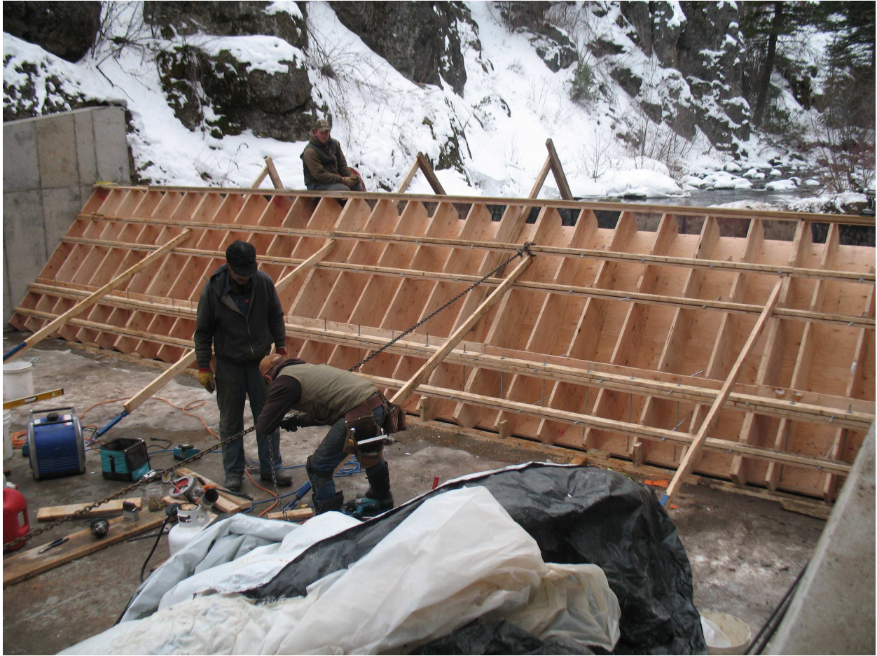
Figure 6. Plywood form for ogee face and constructed wing walls.
