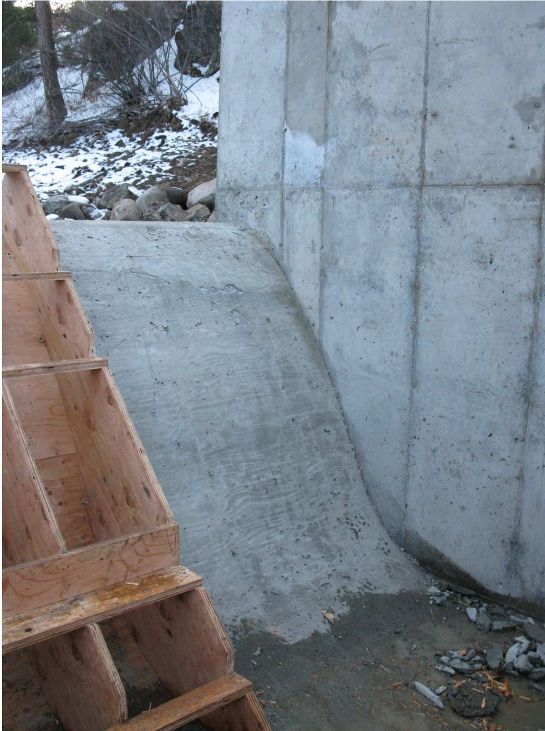
Figure 7. Close up of plywood formed ogee face.
