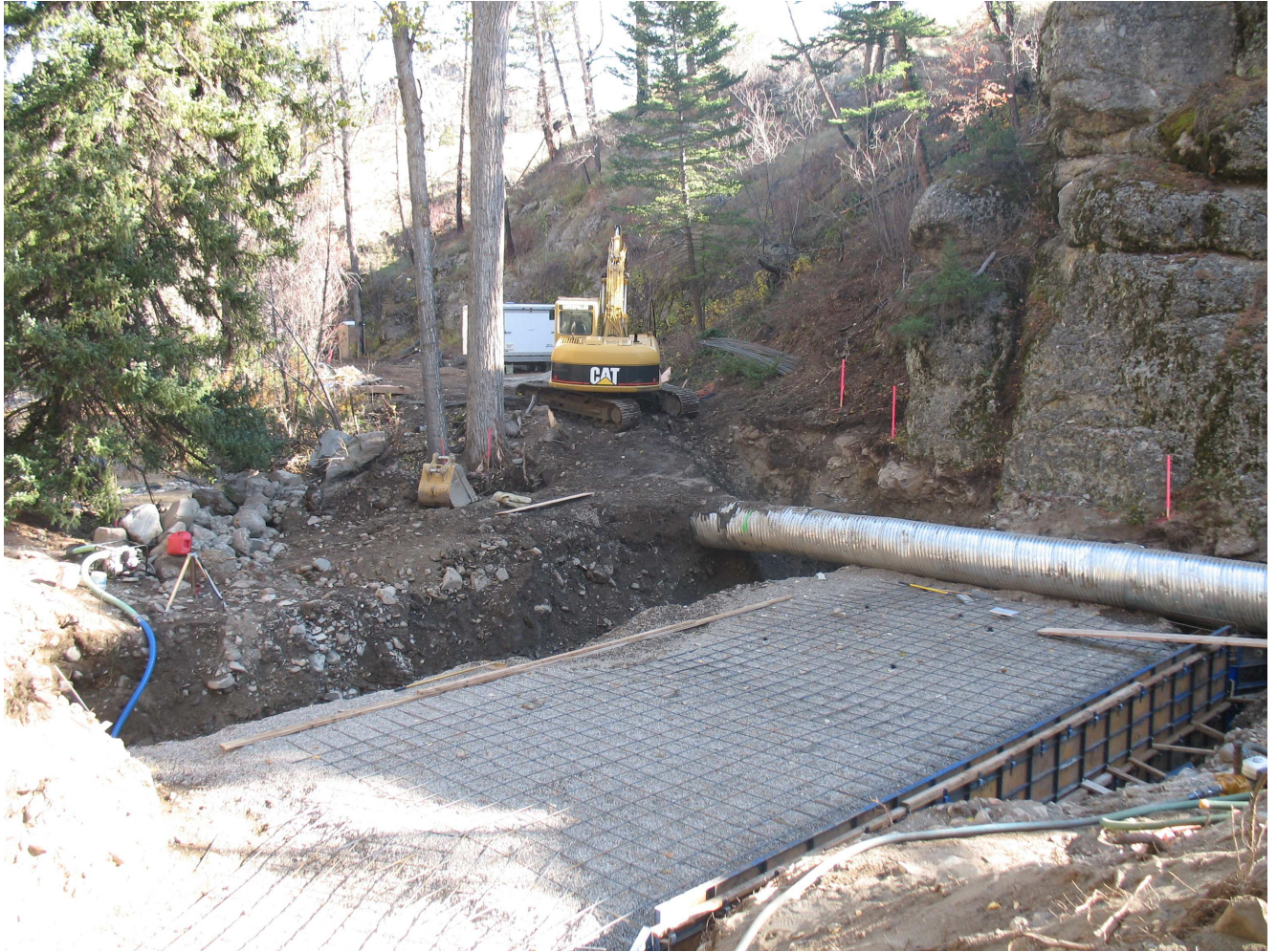
Figure 4. Installation of the foundation of the apron and stream bypass pipe.
