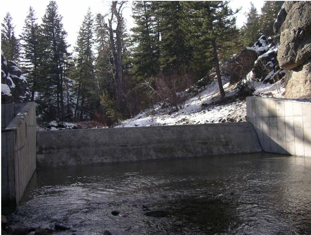
Figure 9. Completed fish barrier.
