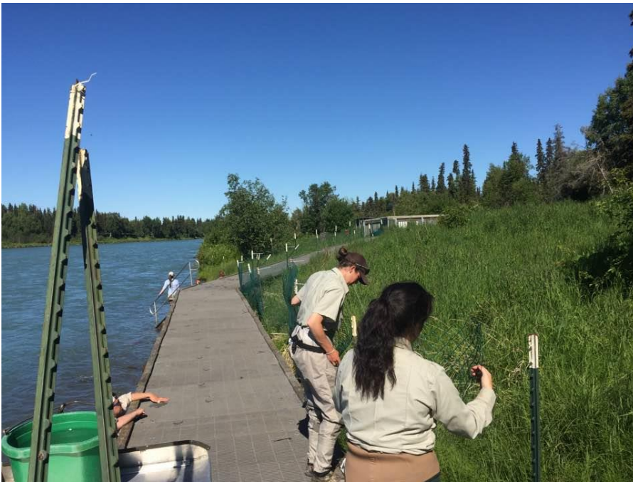
Once T-posts were in place, volunteers helped secure fencing at Moose Range Meadows to protect riparian plants.
