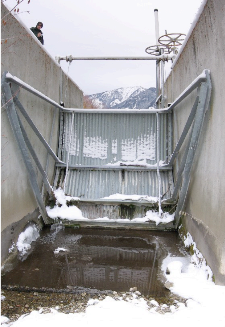
Looking upstream at the barrier headgate at the Georgetown Hydroelectric Diversion during the Winter of 2007.
