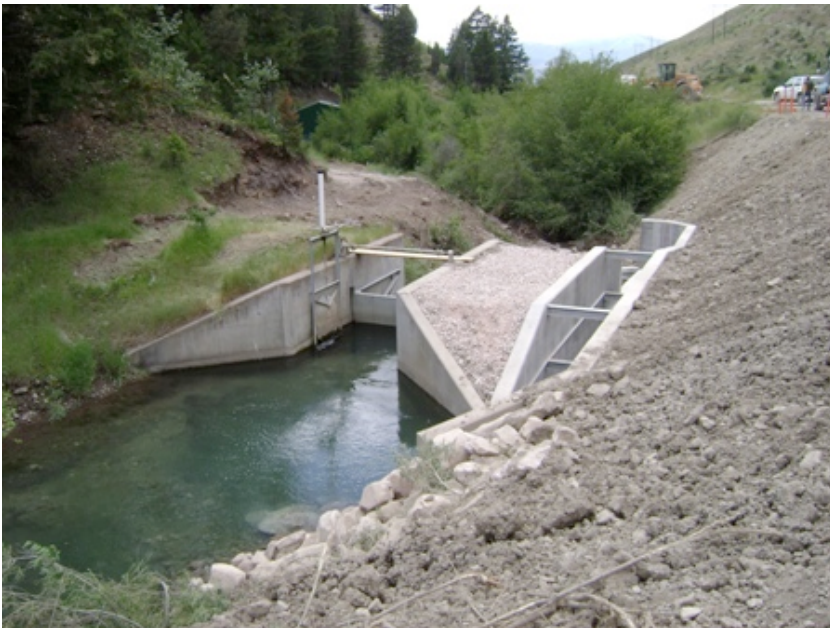
Backfilled fish ladder structure.
