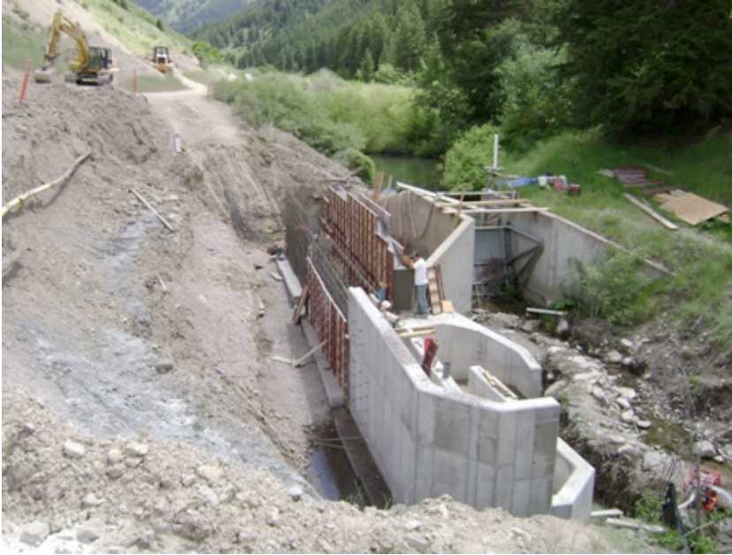
Bureau of Reclamation constructing the Georgetown fish ladder, July 2009.
