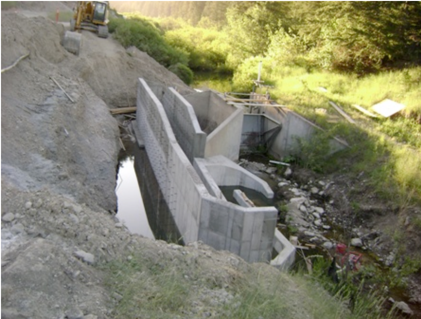
Georgetown fish ladder under construction, July 2009.
