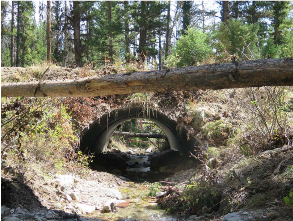
Photos 7-8: Sucker Creek culvert inlet pre and post-project.
