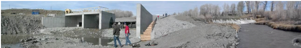
Photo 3: looking upstream at the fish passage ladder on the new Sunshine Diversion.
