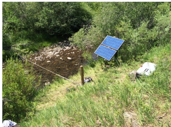
Installed Interrogation site on Canyon Creek.
