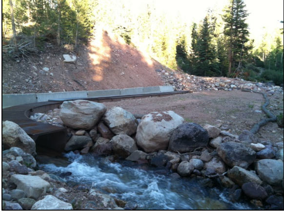
Photo 2. Hovarka Canal fish screen at bypass
