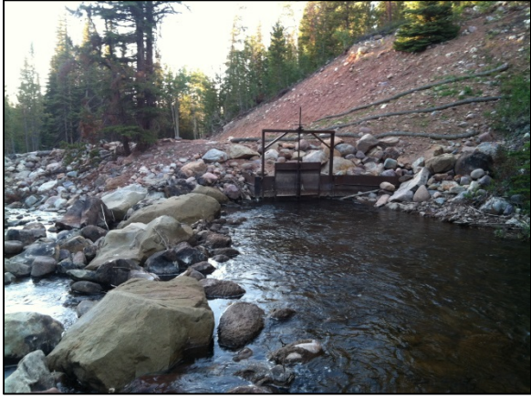
Photo 3. Hovarka Canal new diversion structure.
