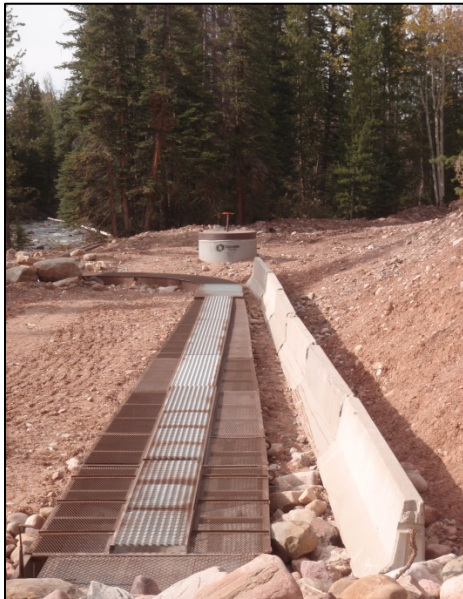
Photo 1. Hovarka Canal fish screen from headgate.
