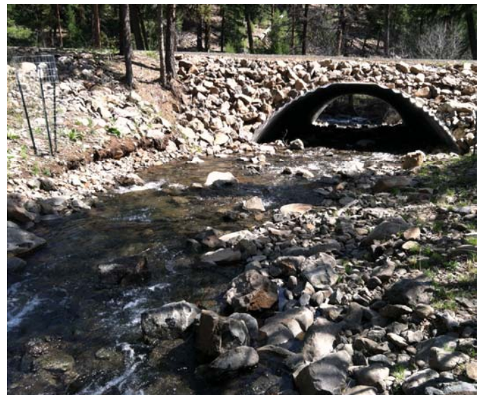
Photo of improved Crazy Creek channel into culvert
