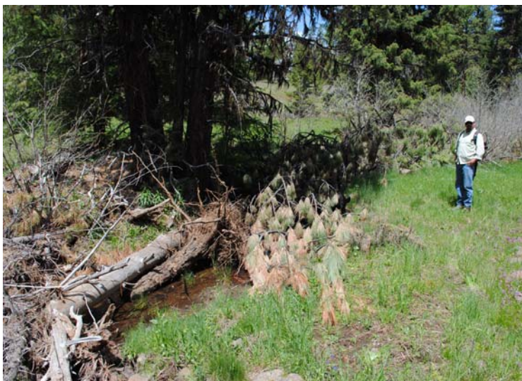
Photo of Photo Monitoring Site 3, After Work Phase II
