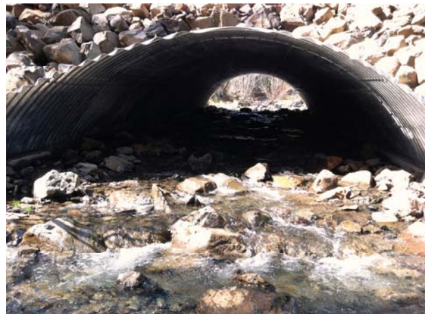
Photo of new bottom arch culvert and sediment
