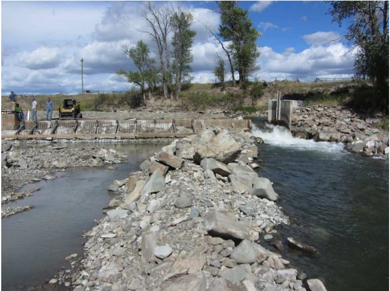
Figure 8. Stage 1, Dewatering and building form for ogee weir face.
