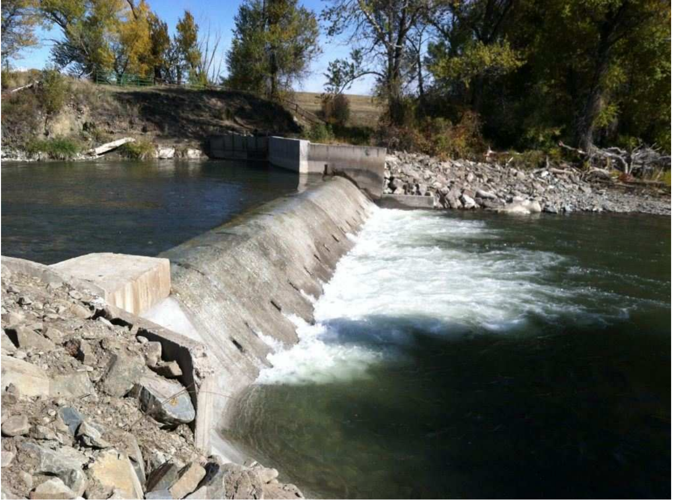
Figure 13. Completed repair and retrofit.
