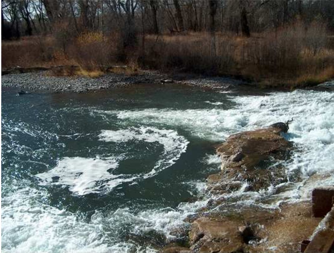
Figure 2. Scour hole and concrete poured to prevent the scour hole from undermining the structure.
