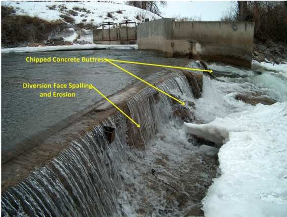
Figure 5. Front wall of the Chadbourne diversion showing erosion and spalling (Allied Engineering 2011).
