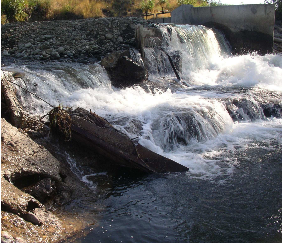
Figure 6. Broken front wall of the Chadbourne diversion and cobble berm placed to check water.
