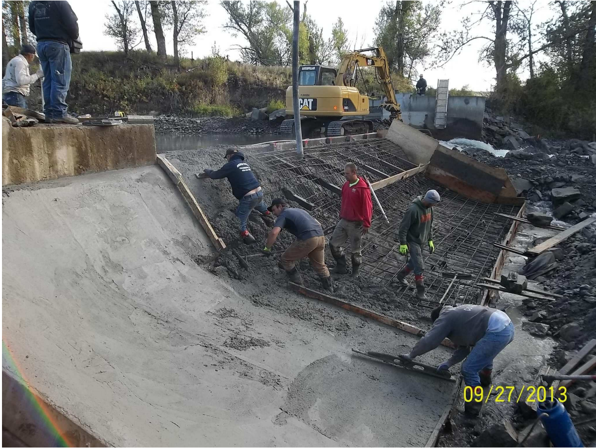
Figure 12. Ogee face being shaped by hand.
