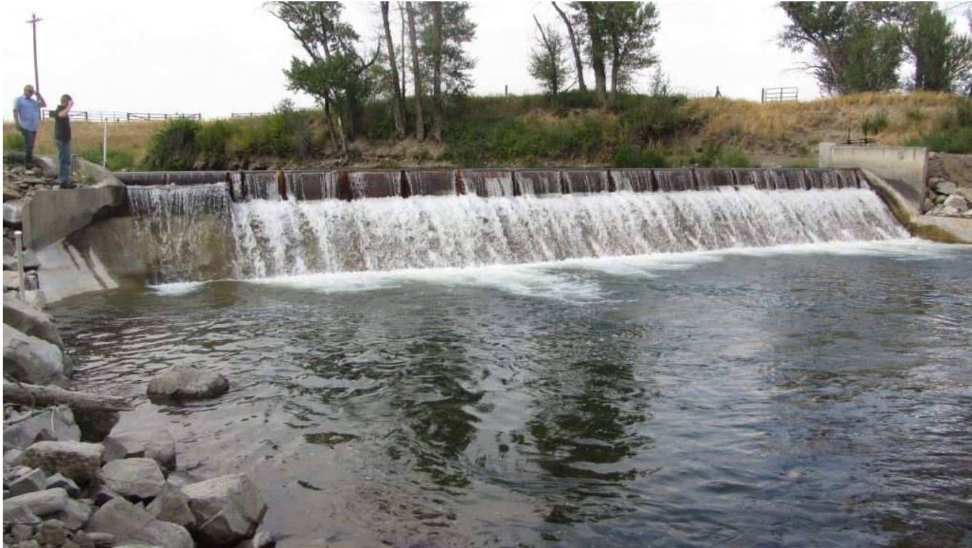
Figure 14. Completed repair and retrofits with the check boards installed.
