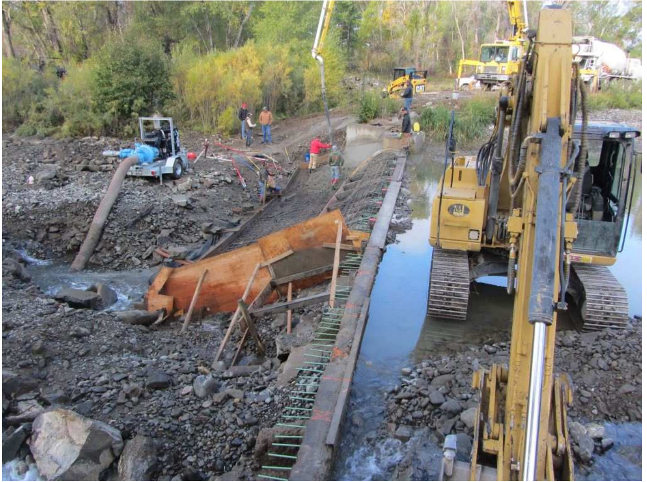
Figure 11. Pouring concrete on right side of diversion.
