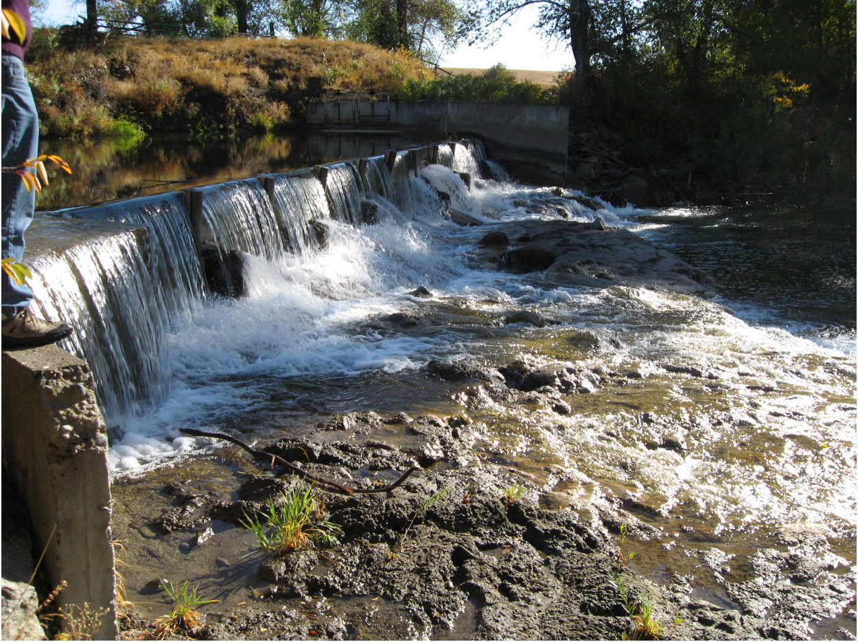
Figure 3. Irregular concrete slab that decreased the leap height, and provided roughness
