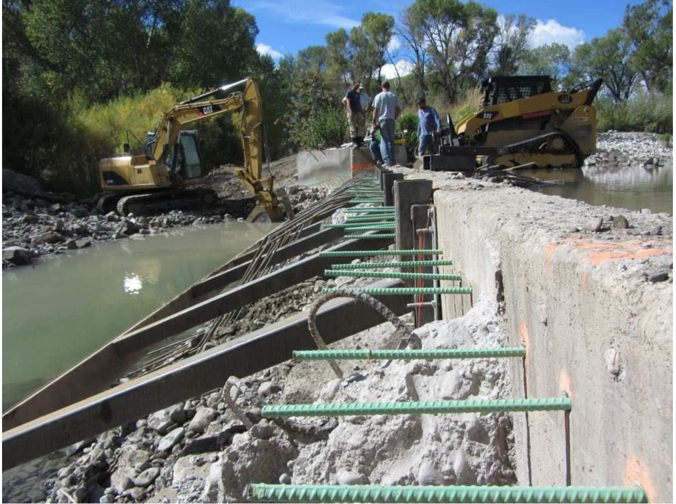
Figure 9. Installation of pipes to hold vertical planks that hold the check boards in place.
