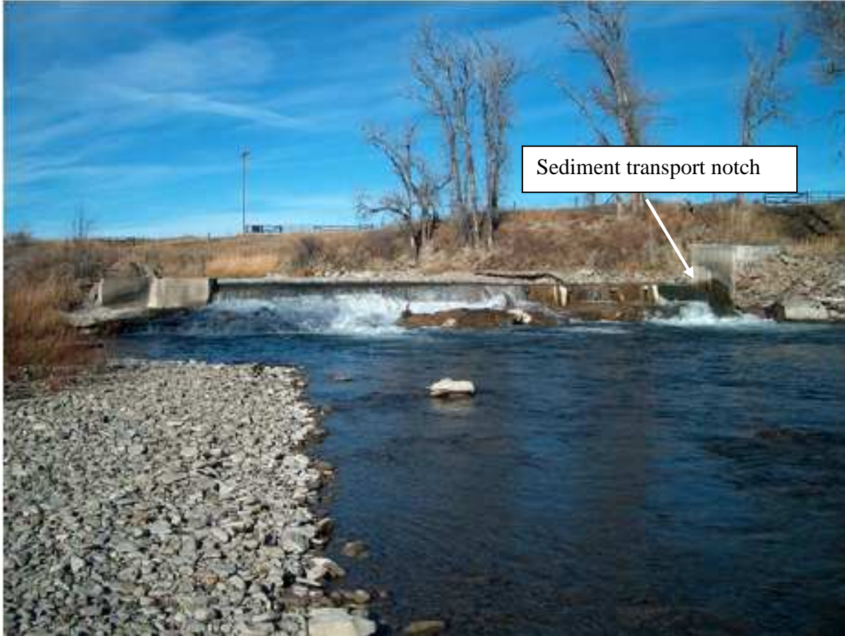
Figure 4. View of Chadbourne diversion looking upstream showing sediment passage notch.
