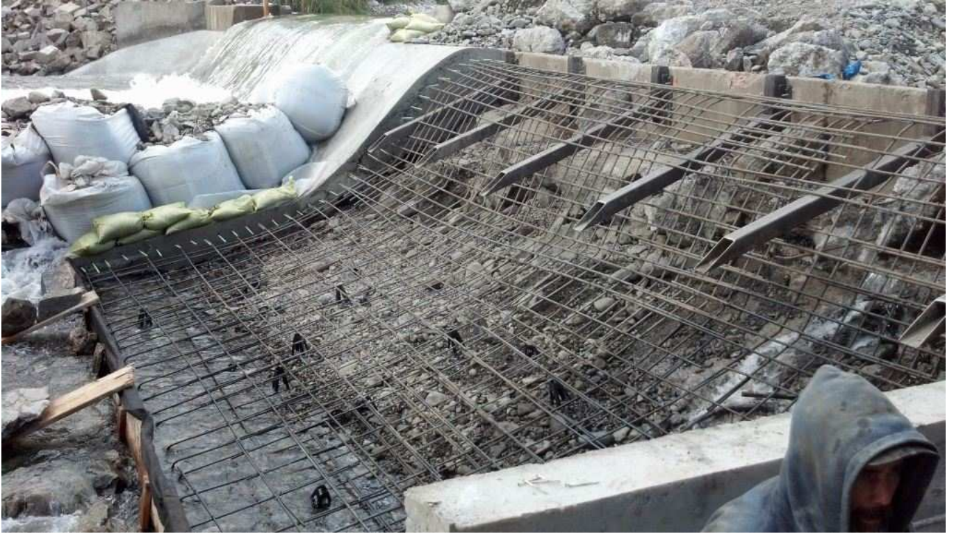
Figure 10. Close-up of metal frame for ogee weir.
