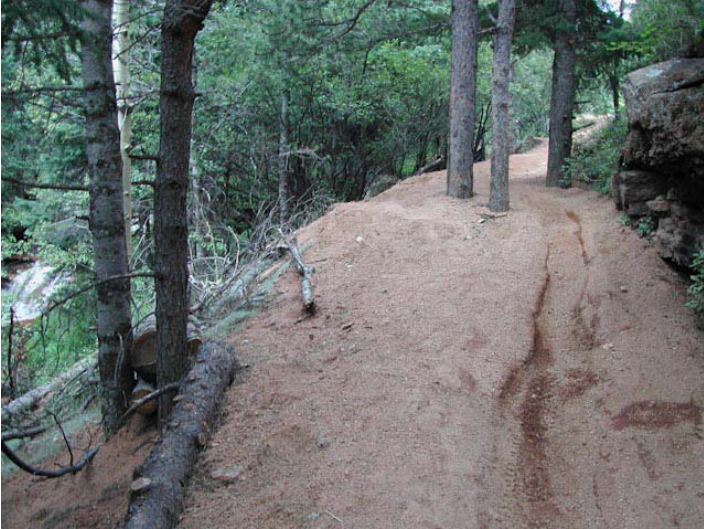
Img. 15: BEFORE. Trail is unnecessarily wide and outslope is unstable.
