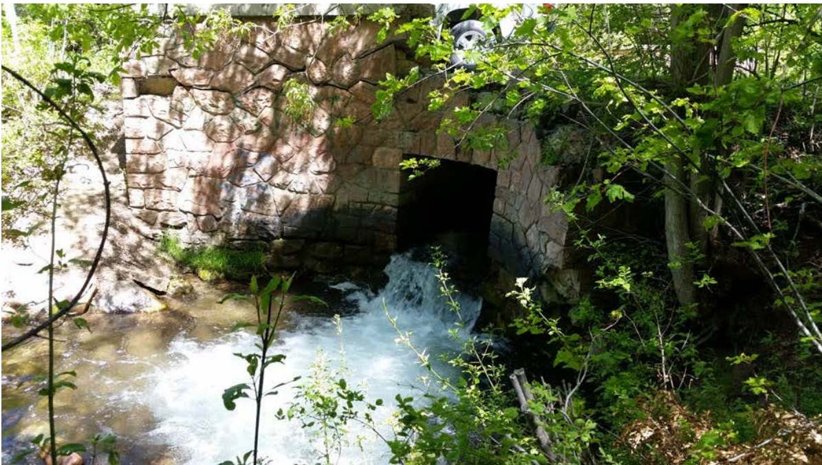
Outlet of rock culvert
