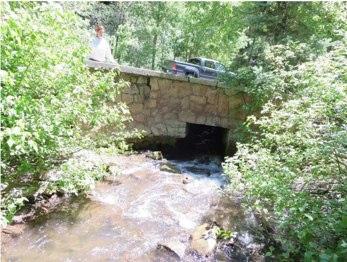
Inlet of rock culvert similar to the one that will replace the fish passage barrier on Mill Creek
