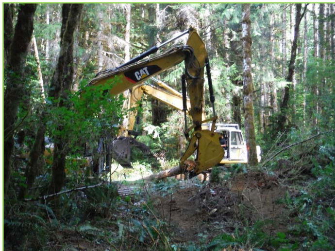
Randy & Nick/JTS - working 2 excavators
