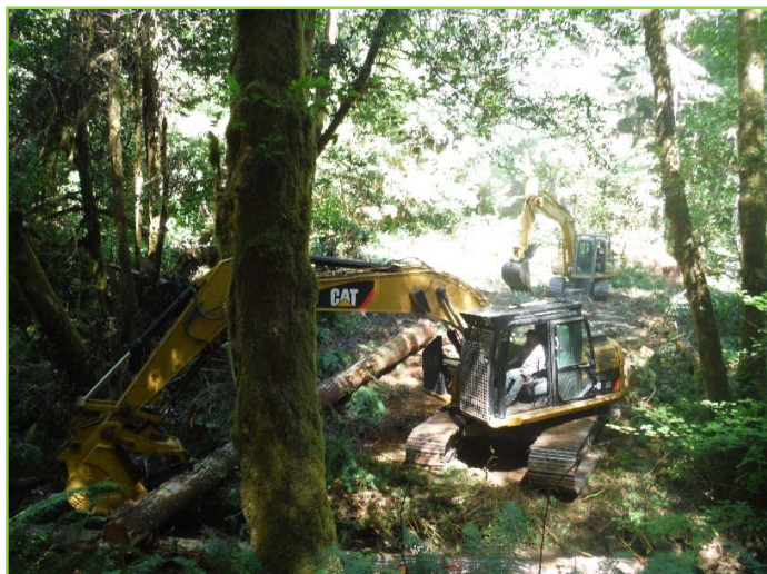
Randy & Nick/JTS - working 2 excavators
