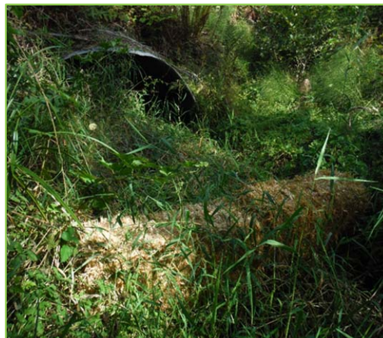
Sediment controls were placed throughout the project
