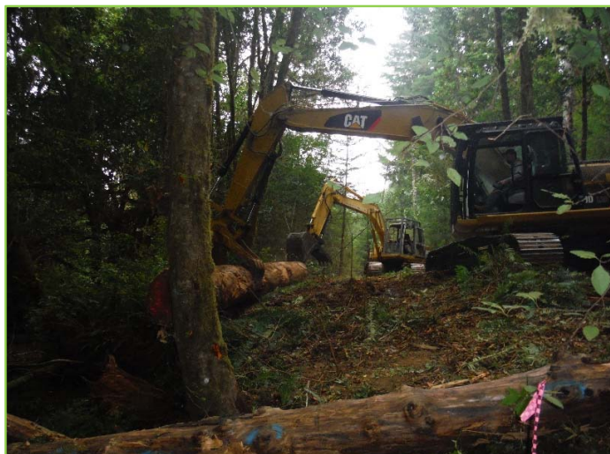
Randy & Nick/JTS – working 2 excavators
