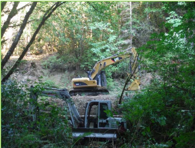
5 excavators were used on-site
