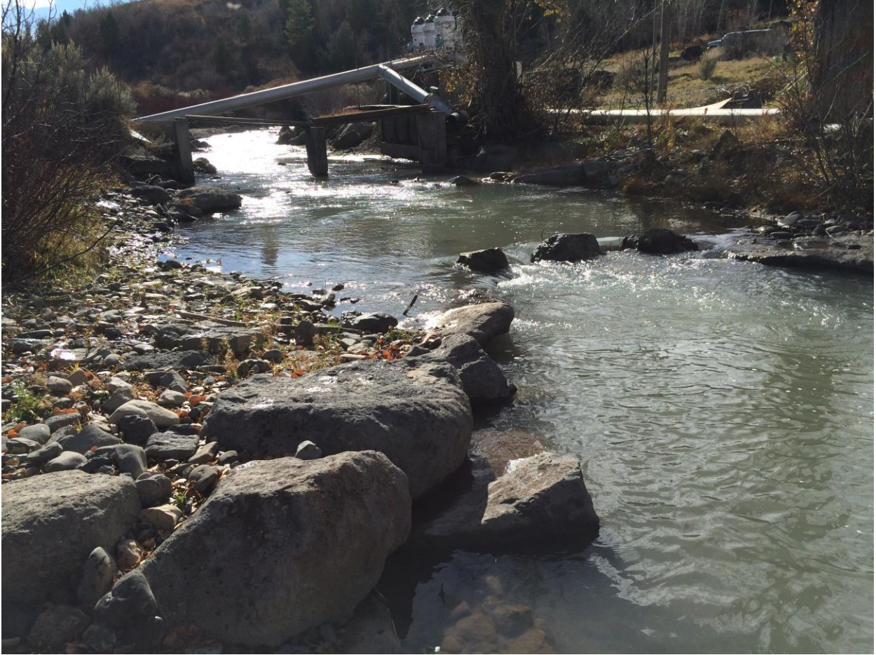
Figure 3. Upstream view of two of the rock weirs and submerged check dam slab.
