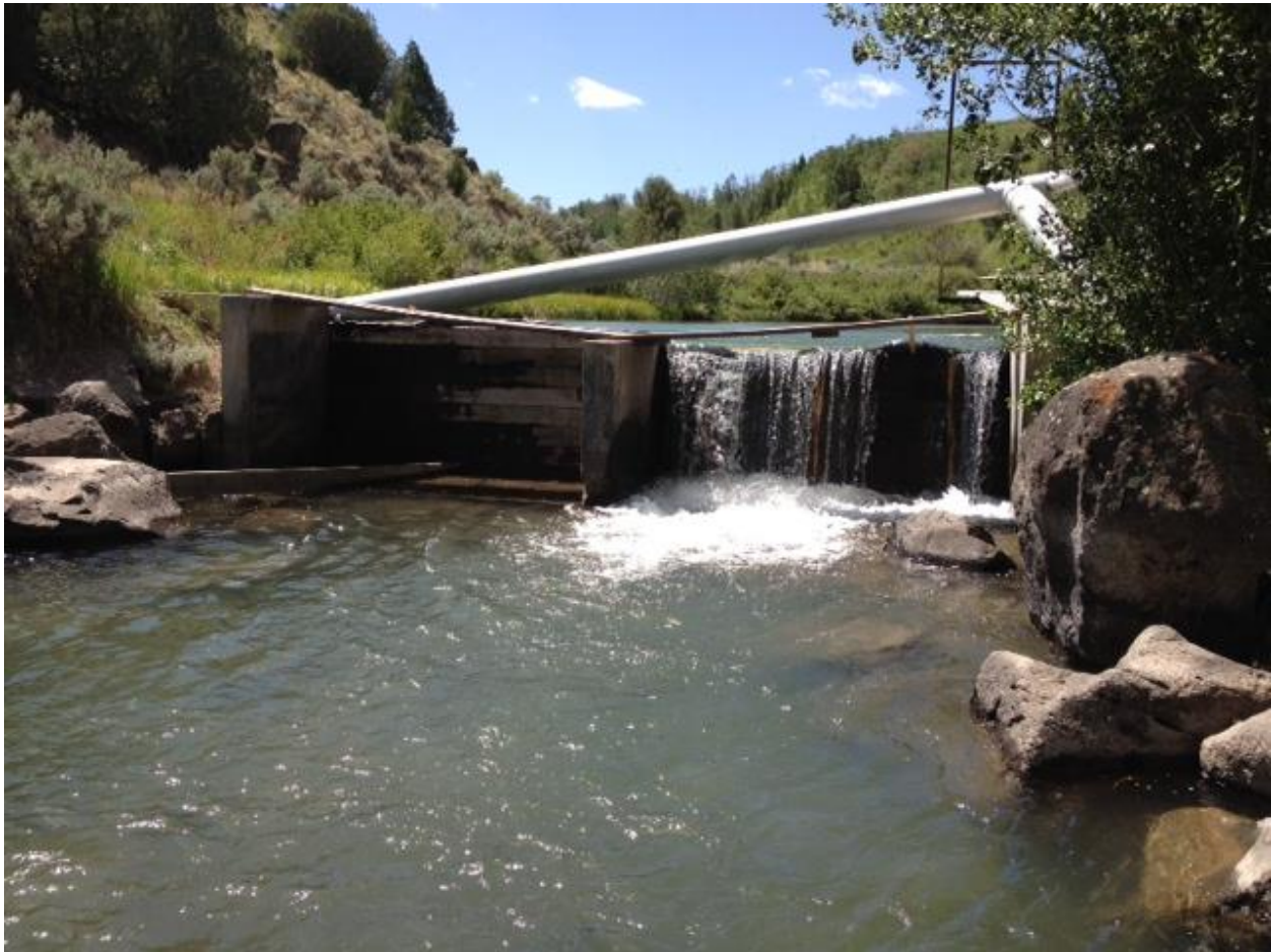
Figure 2. Pre-project photo of the check dam
