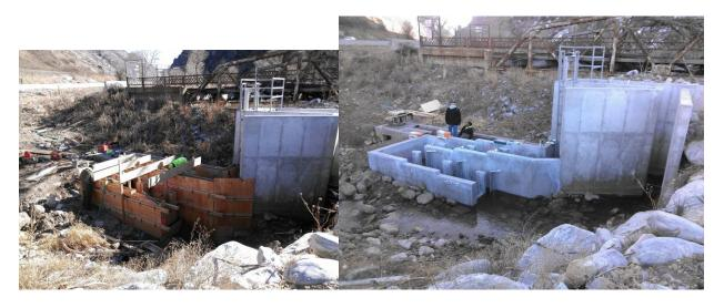
New fish ladder at the Mouth of Weber Canyon. During 2013 over 1100 fish of all species moved through this fishway around the diversion dam. Biologists observed a high velocity bottleneck in the fishway at high flows, when fish typically move the most. The final concept was a fish ladder that is active only at high flows, which enters back into the top of existing fishway.
