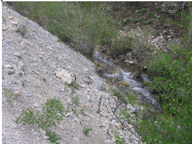
Concern: Slag-laden Georgetown Road adjacent to, in, or over Georgetown Creek.
