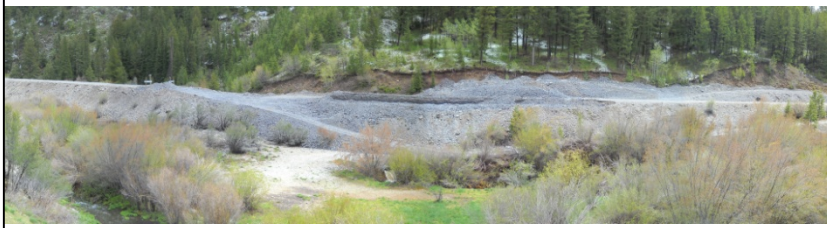
Upper end of project area taken near Church Hollow. One of the remaining perched culverts, to be removed in Phase IV is located in the center of the photo.
