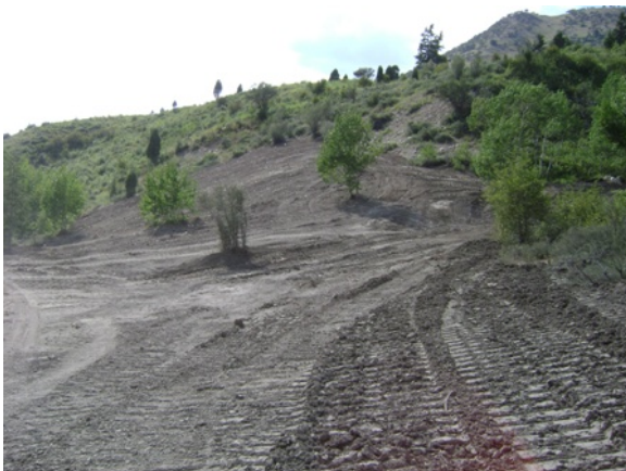
One of the upland deposit sites. We chose excavated areas to spread the road fill material and cover it with soil. These areas will be hydromulched with native grass seeds this fall.
