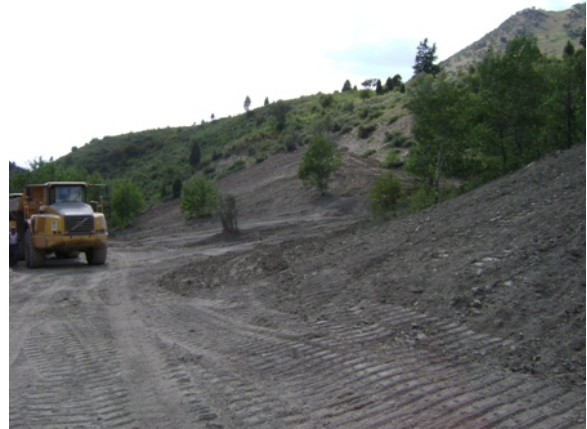
Another upland deposit site ready for planting.
