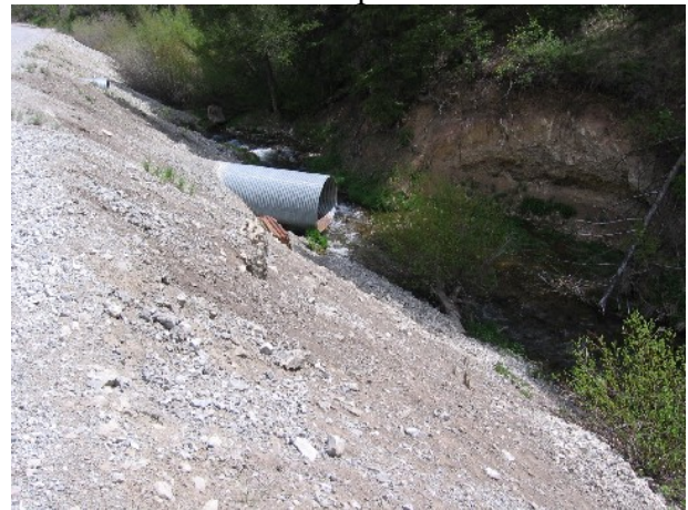
Concern: In addition to Georgetown Road encroaching upon the stream and its floodplains, it presents significant migration barriers to upstream-migrating fish. Capurso prepared an environmental assessment during the winter of 2007-8 for the removal of the road from the stream and its floodplains. Close coordination between the Forest Service, the City of Georgetown, Idaho Department of Environmental Quality, and U.S. Environmental Protection
