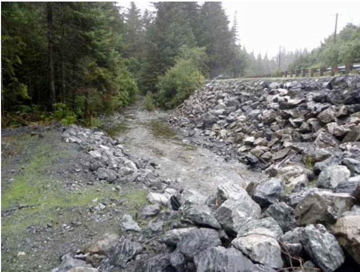
Figure 5: Looking downstream Eccles Creek on the downstream side of the culvert.
