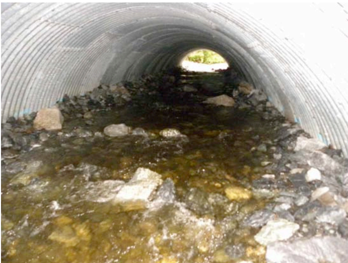
Figure 8: Looking upstream at the downstream side, inside the Eccles Creek culvert.
