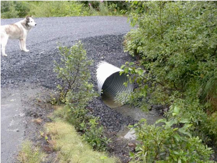
Figure 13: Looking upstream at the downstream side of the Bartley driveway culvert. This ditch now drains stormwater from the City Baler.
