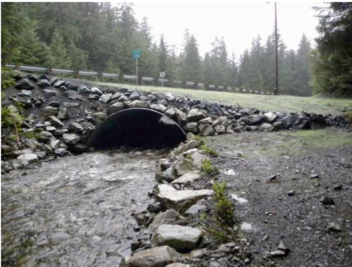
Figure 4: Looking downstream at the upstream end of the new Eccles Creek.
