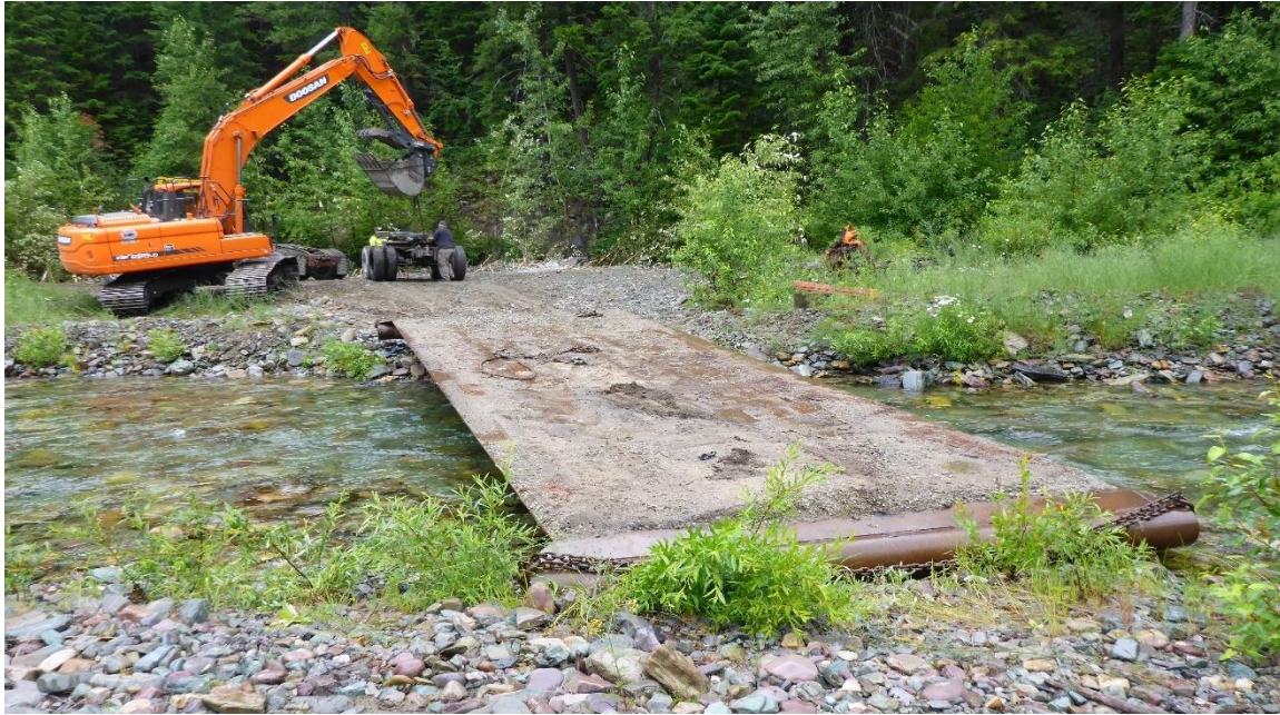
Figure 4.0 Temporary bridge built and installed for the Miners gulch reach restoration.
