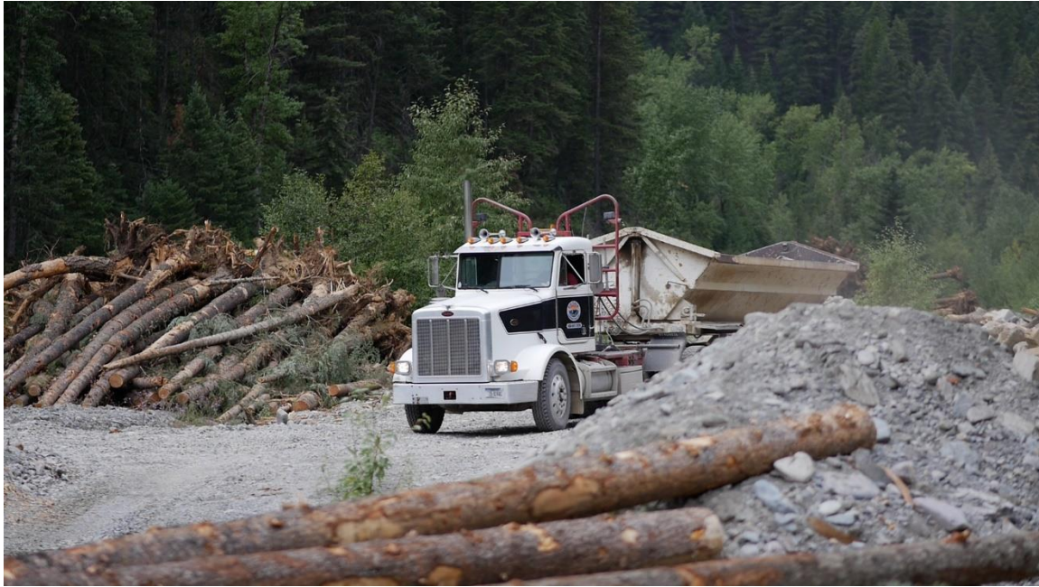
Figure 4.2 Large wood stockpile at staging area within the immediate project work site.
