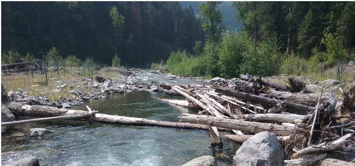
Figure 7.4 Example of the large wood additions within the project subsequent two runoff cycles in the Vermilion River (white wood).
