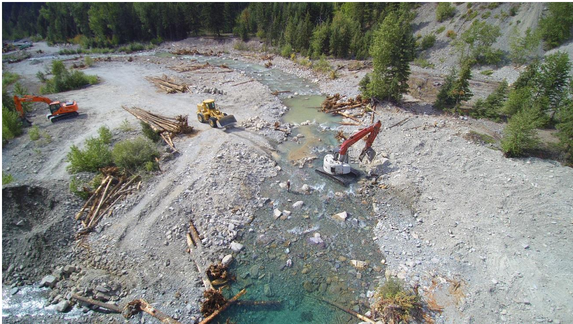
Figure 4.1 2016 construction activities during the Miners gulch reach restoration.
