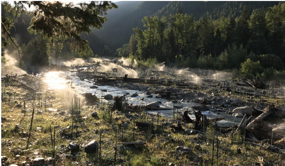
Figure 5.0 Irrigation of the planted riparian vegetation with fenced enclosures on the constructed floodplain.
