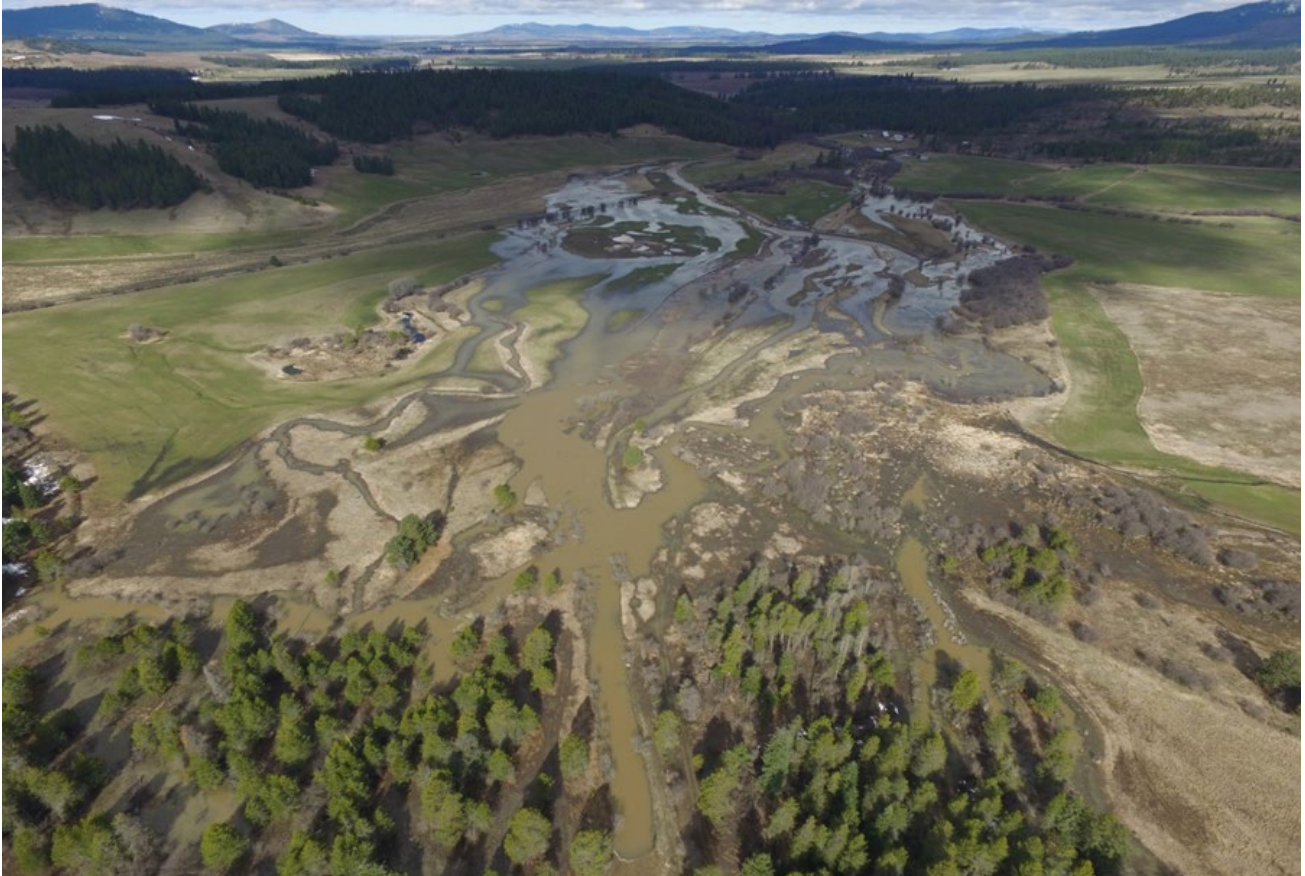
Picture 4. After picture of project site during runoff event at approximately 300cfs, March 2017.
