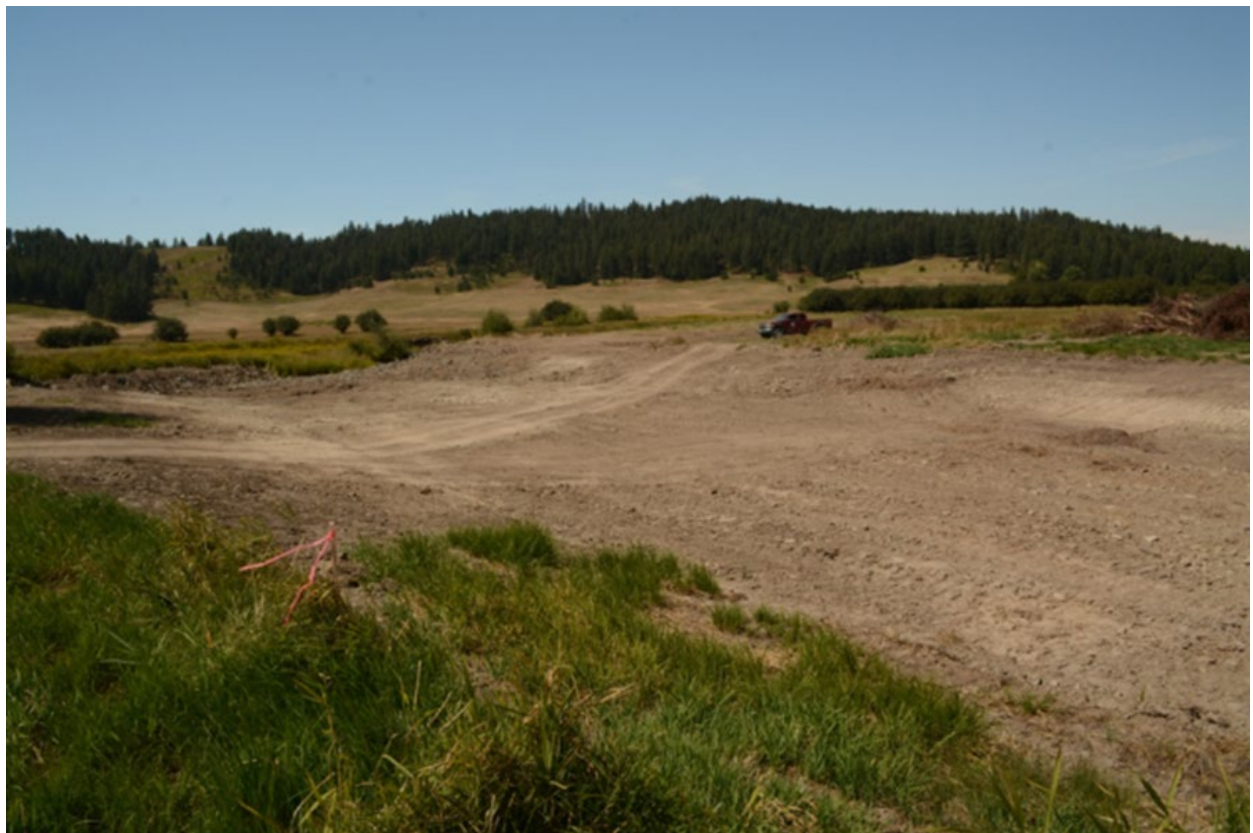
Picture 2. Constructed relief channel Aug, 2016.
