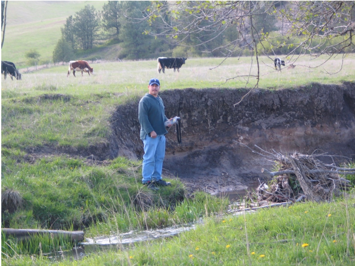
Picture 5. Portion of the channelized stream within project site prior to restoration actions. Photo taken during early summer of 2010.
