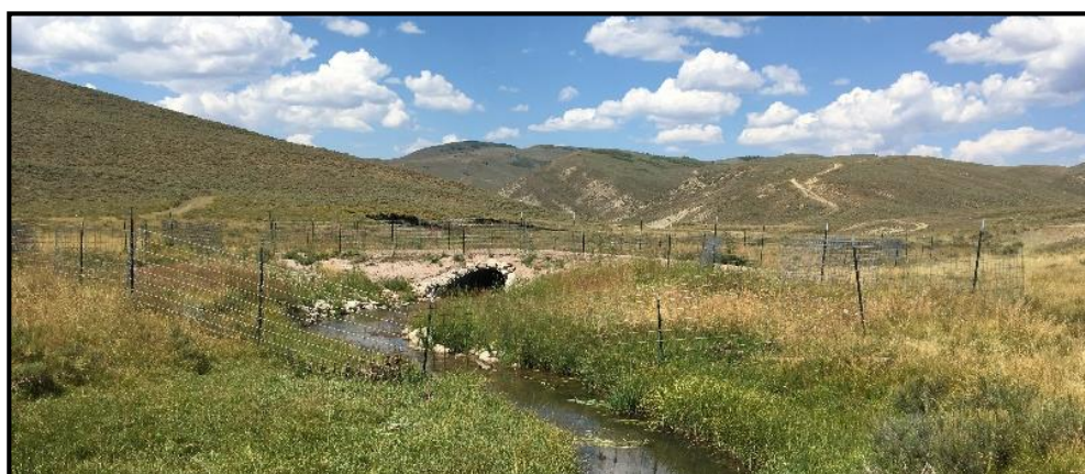
A vehicle ford on Little Muddy Creek was replaced with a bottomless arch culvert to improve stream function and road safety at this site.
