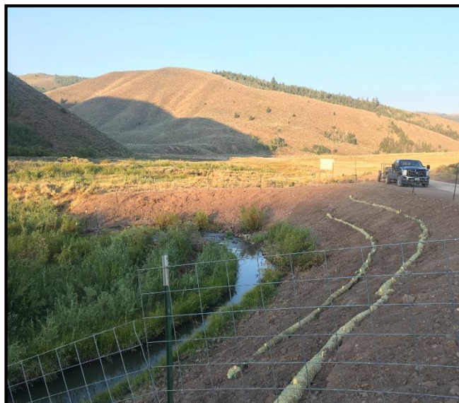
Photos from before (left) and after (right) bank re-sloping and construction of a bankfull bench to reduce sediment inputs from a large eroding bank.
