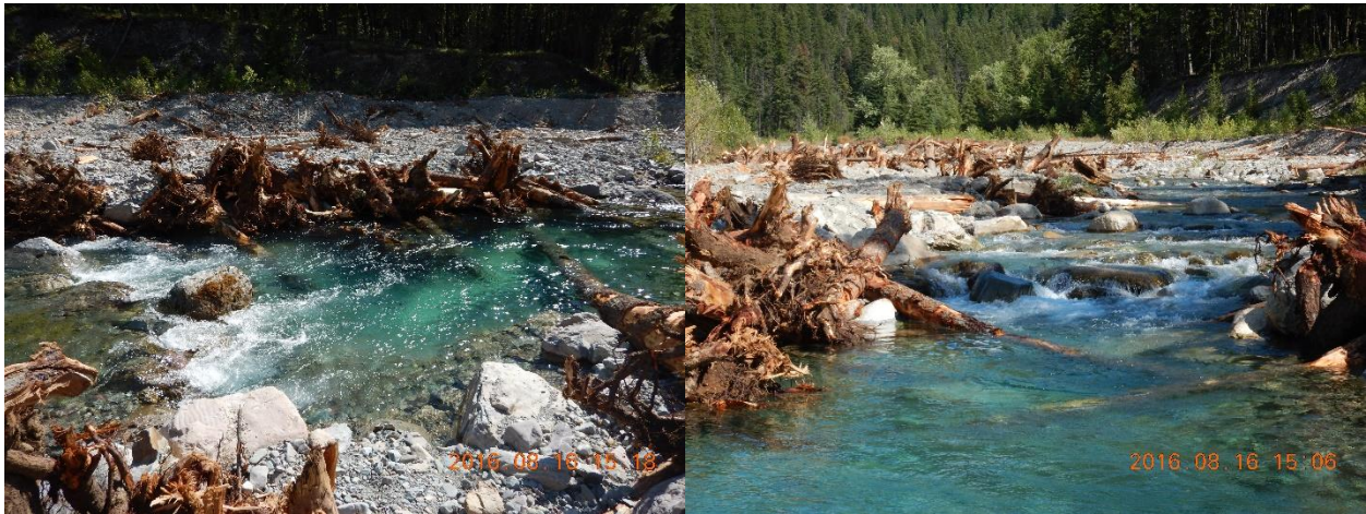
Figure 3. Completed channel reconstructed with rock and log structures and newly created pool habitat in the Miners Gulch reach of the Vermilion River.
