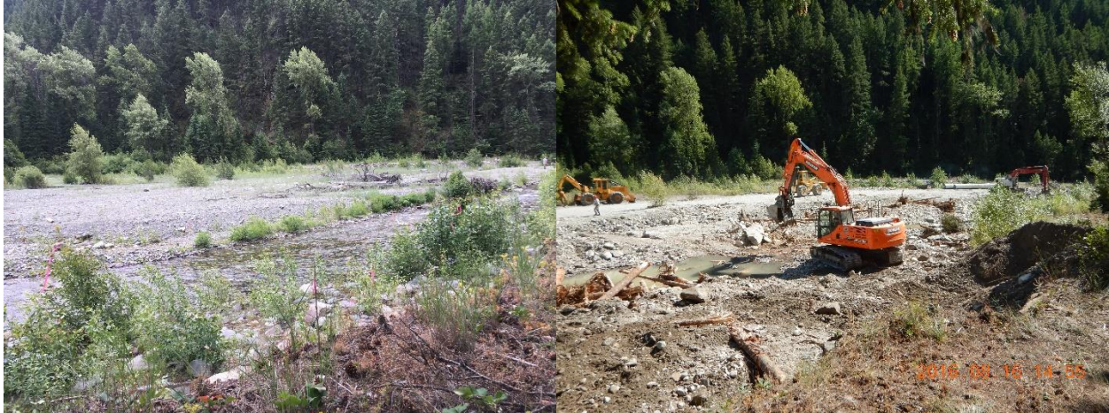
Figure 1. A section of the Miners Gulch Reach of the Vermilion River pictured prior to channel reconstruction is shown on left and excavator reconstructing the same section is on the right.
