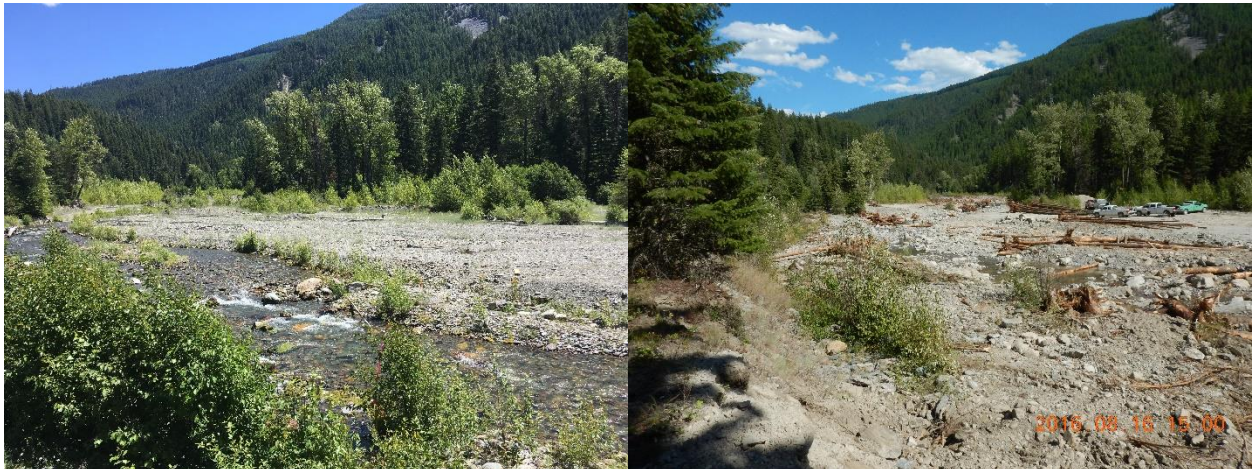
Figure 2. Pointing upstream from the same location where photos were taken in Figure 1, the left shows the stream channel and floodplain prior to channel reconstruction work and the right shows the stream channel and floodplain during the middle of implementation.
